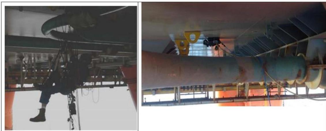
*Fig. 1 Shows a comparison of the worker driven inspection and the equipment required to do so (left), vs. the robotic crawler driven inspection (right). Both methods are carrying out an inspection on a very difficult to access underside area of an oil rig [14].*
