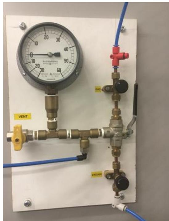
**Figure 3-25.** Gas control devices.
