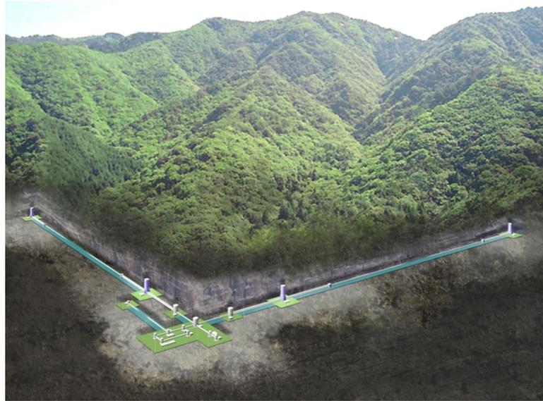
Figure 1.7: Artistic impression of the underground interferometer in the Kamioka mine. The KAGRA detector consists of a dual recycled Michelson interferometer with arm lengths of 3 km. The detector operates at cryogenic temperatures hence utilises sapphire test masses unlike the fused silica components within the detectors operating at room temperature. Illustration reprinted from [39].
