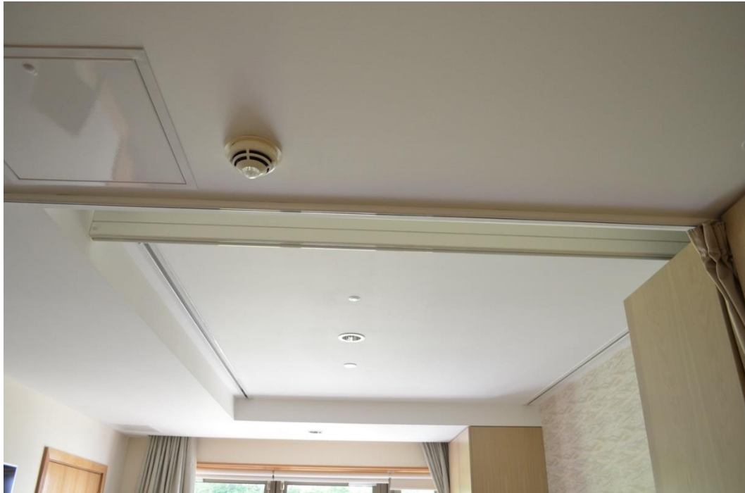
Figure 9-15 Integrated hoist concealed within the ceiling design.
