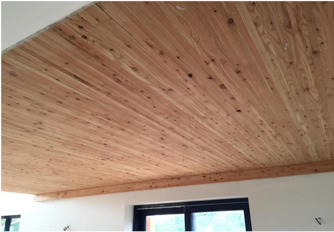
**Figure 9-7: Intermediate DLT floor deck 1.**
