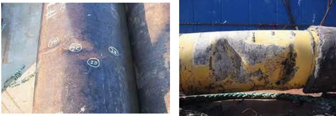
**Figure 3.1** The plain dents on the offshore cylindrical structures (Alexander and Brownlee, 2007; Macdonald et al., 2007)
