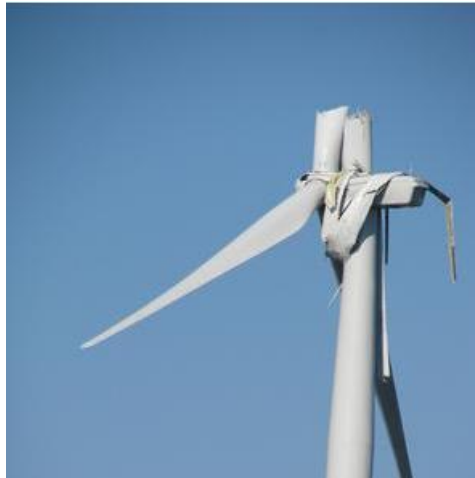
Figure 1.2 Wind turbine blade broken [5]
