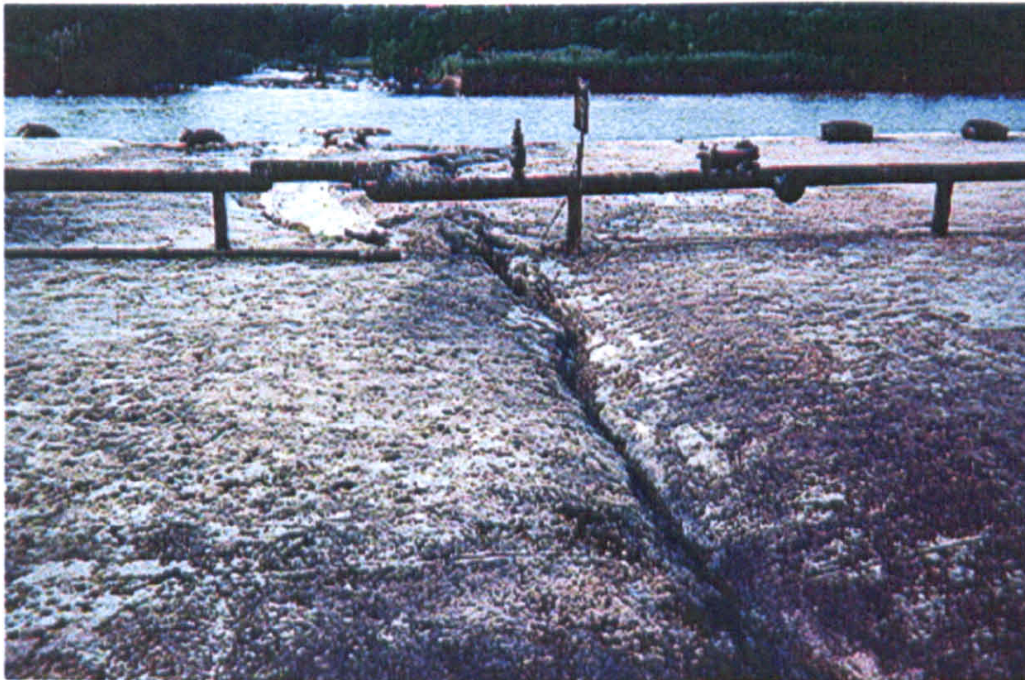
Figure 1.3: Deck plate buckled on BUFFALO 286
