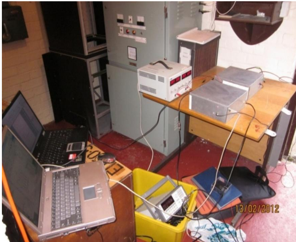
Figure D-15 PDDN on-site trial @ 33/11 KV Substation, Edinburgh
