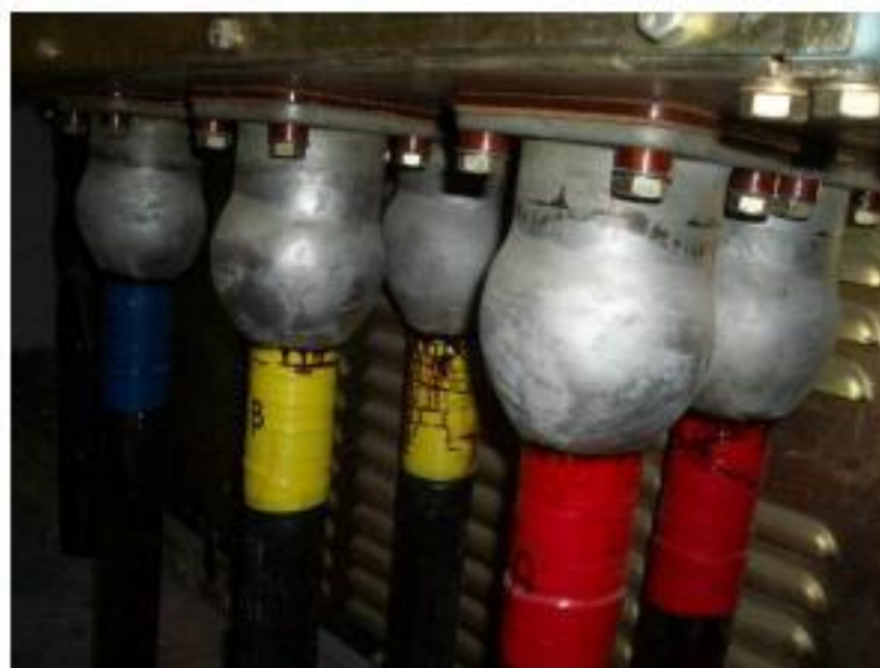
Figure 2-29 Solidly bonded termination
