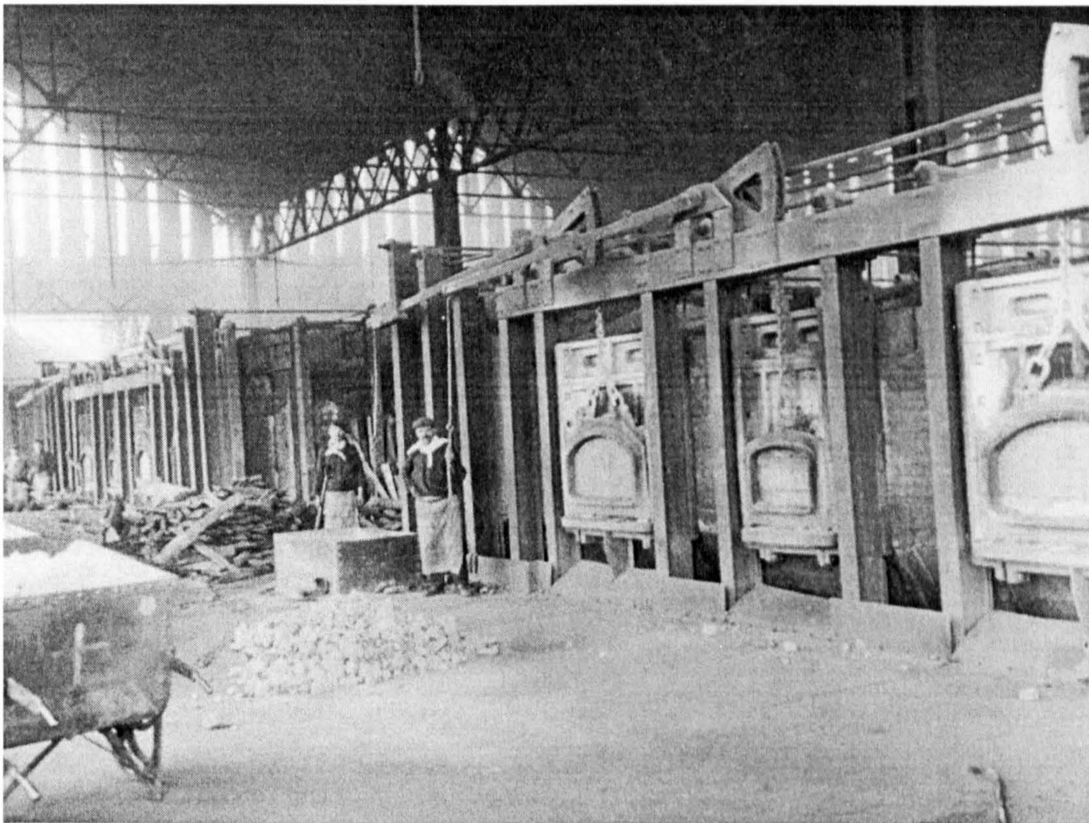
Figure 19. Charging side of 50-ton Siemens furnaces at Clydesdale, c1905.
