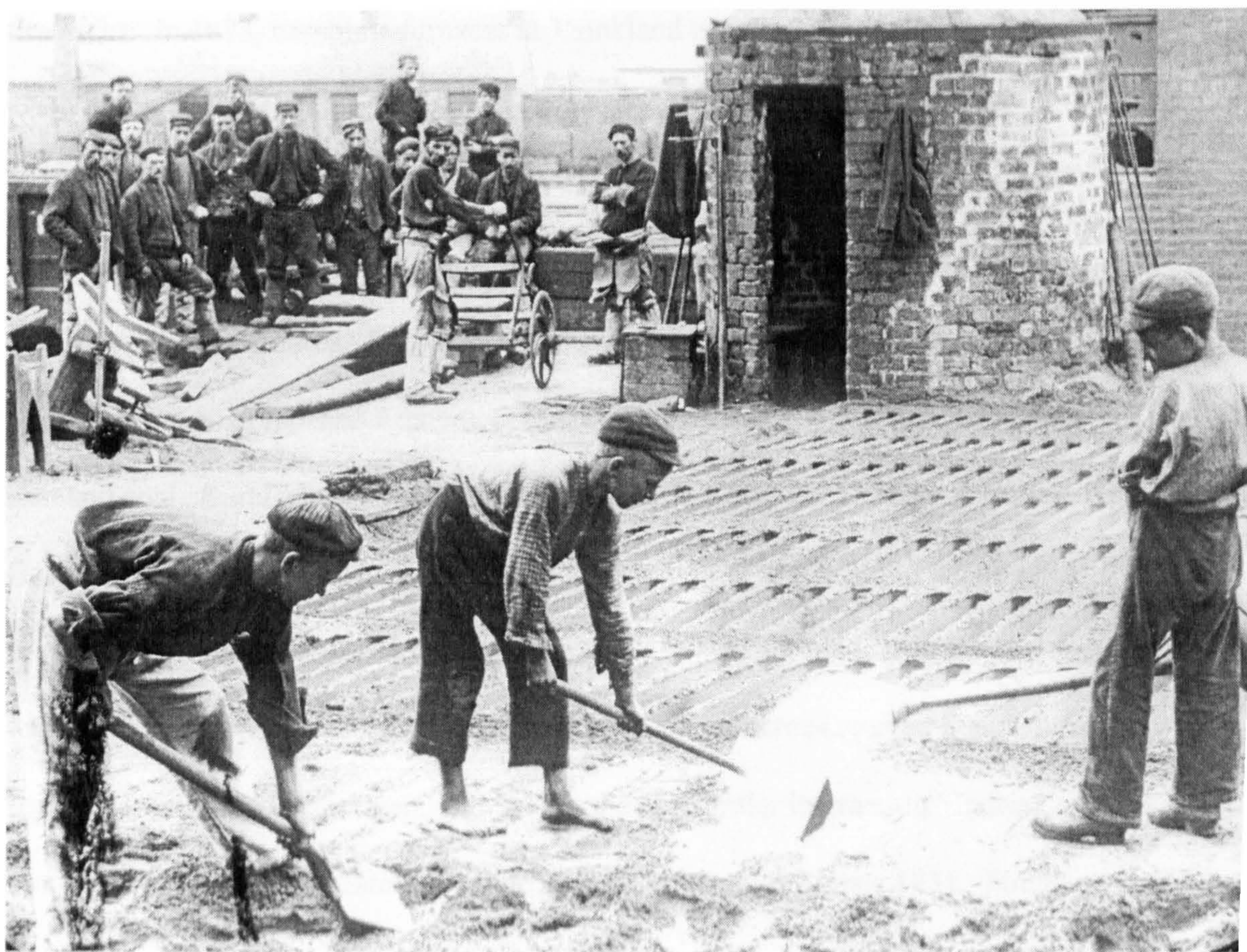
Figure 12. Boys making pig-beds, Coltness, c1890. One boy (right) dampes the sand whilst others shape the pig-beds that were filled with molten iron. Despite the danger, one boy is bare-foot.
