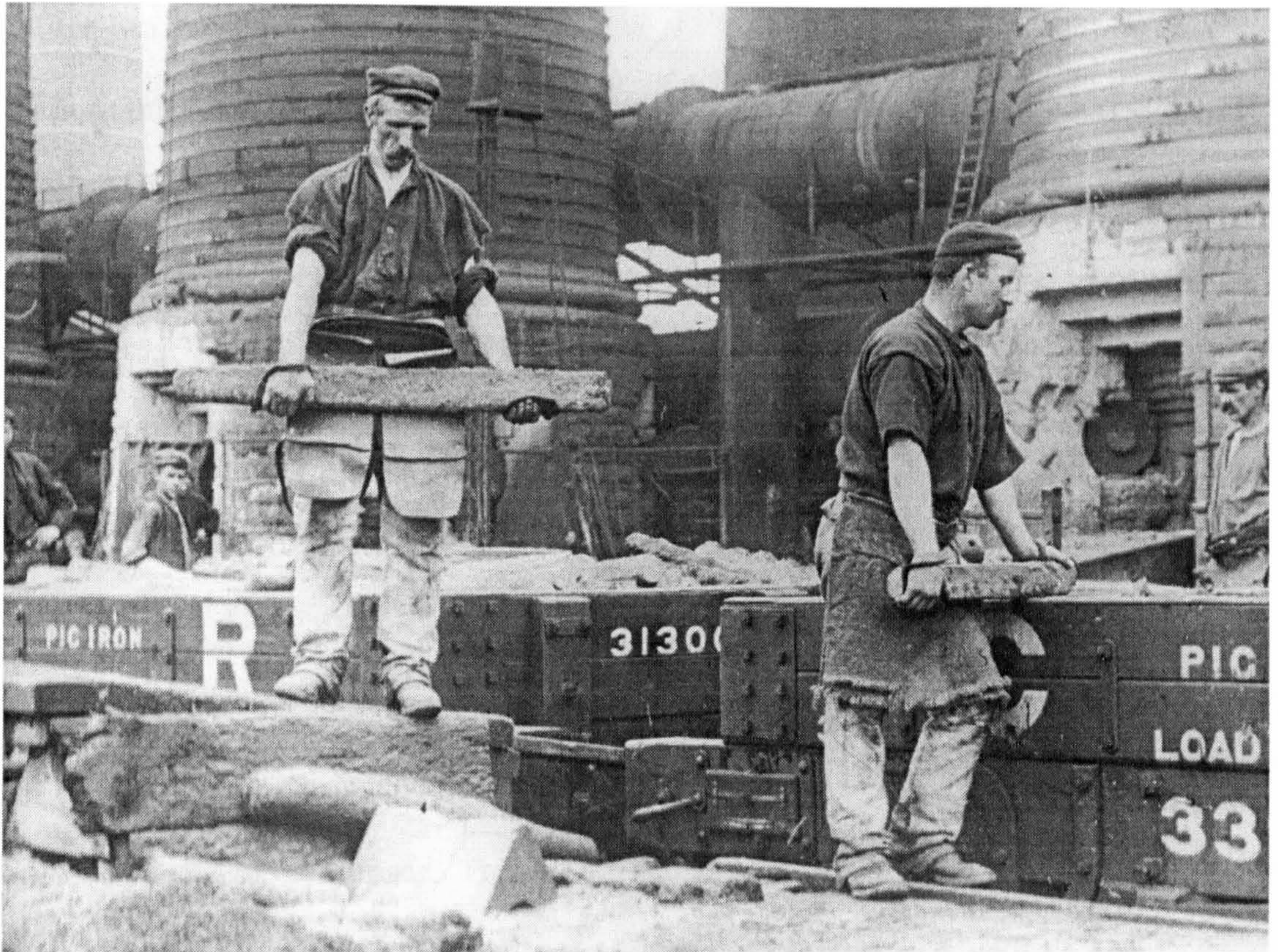
Figure 11. Pig lifting at Coltness, c1890. Each pig weighed over 1 cwt. Dropping onto the ‘v’-shaped stone fractured the pig, which was then loaded into wagons for transportation. Although the pig-lifter’s hands and legs are protected by leather, the exhausting nature of pig-lifting is apparent.
