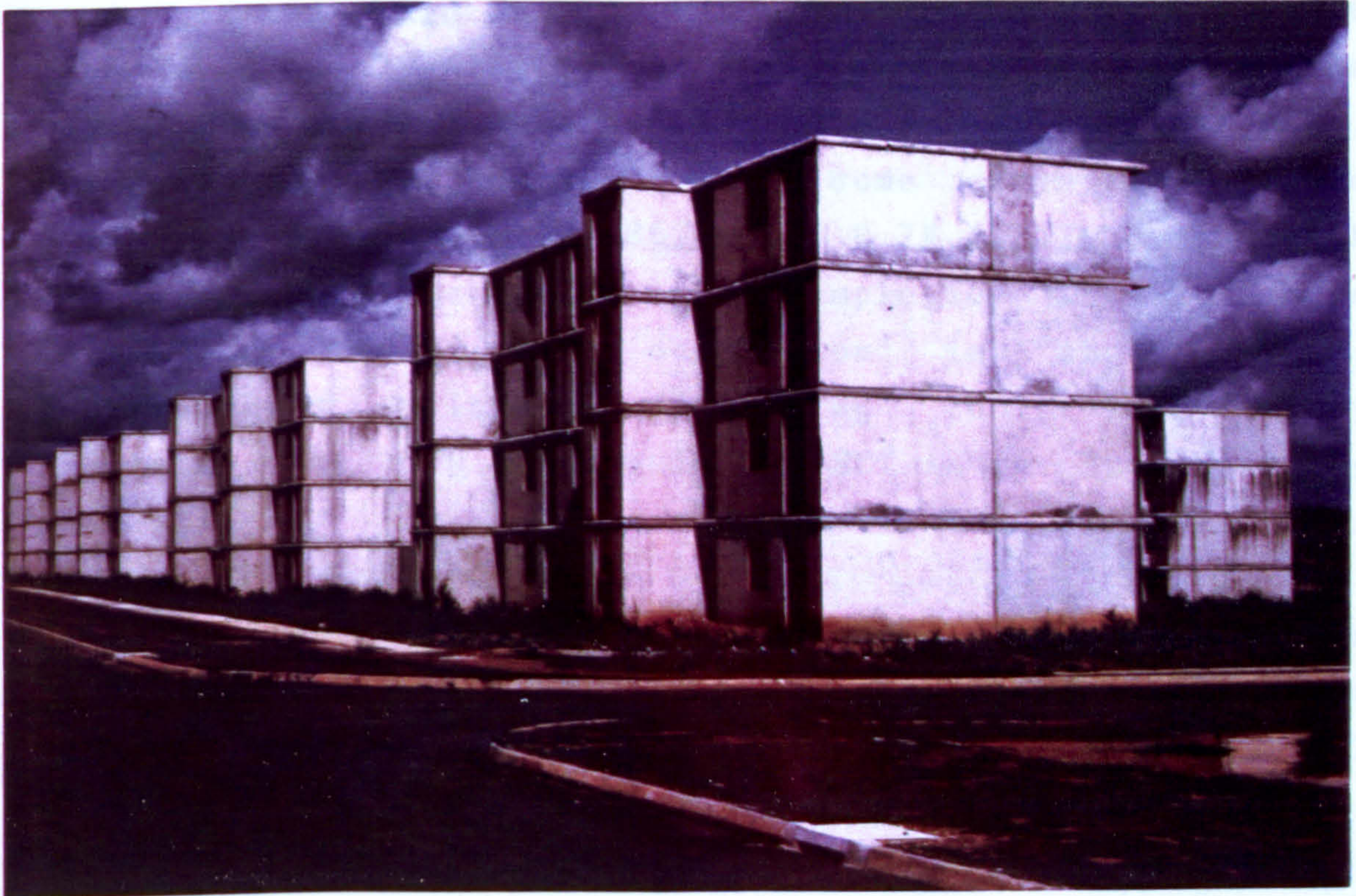
Figure 5.7. Blocks of Flats - Erected with Prefabricated Components, Abandoned Due to Lack of Appropriate Building Fixtures - Garki District
