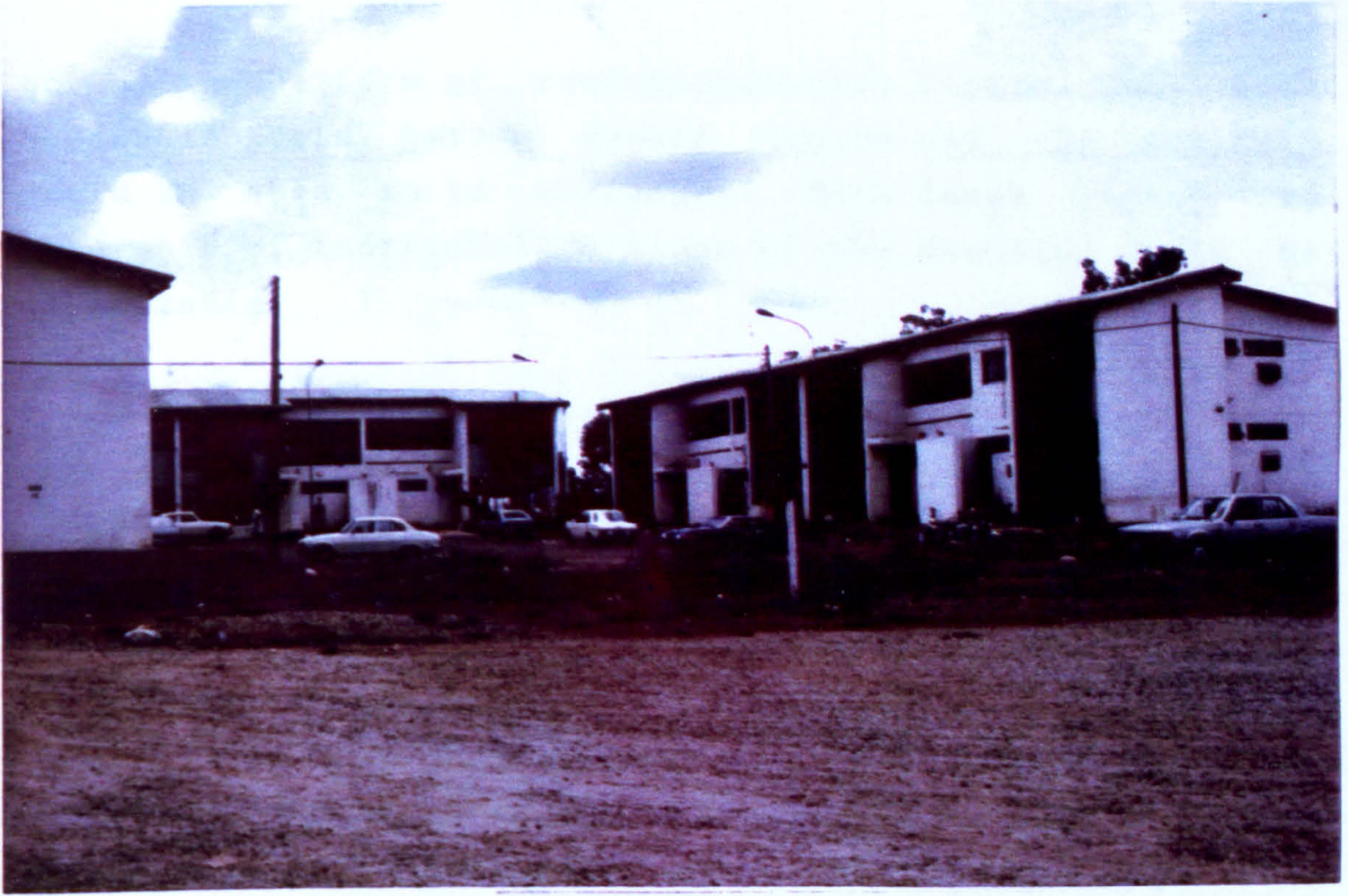
Figure 4.3: Three Bedroom Semi-Detached Houses, Garki District
