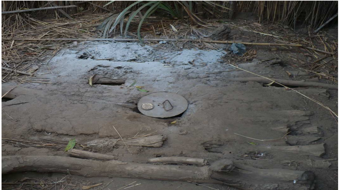
Figure 4: A traditional pit latrine showing logs placed over the pit covered by earthen mud in Lungwena, Mangochi District
