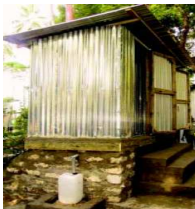
Figure 8: The Skyloo with urine diversion toilet in Mombasa, Kenya
