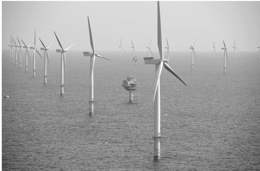
Figure 2.3: Wind turbines of the Danish three-bladed concept at Sheringham Shoal [3]
