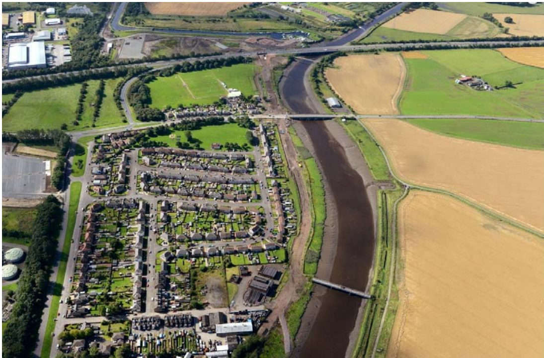
Figure 1.4 A photograph showing the new canal stretch alongside the River Carron 13
