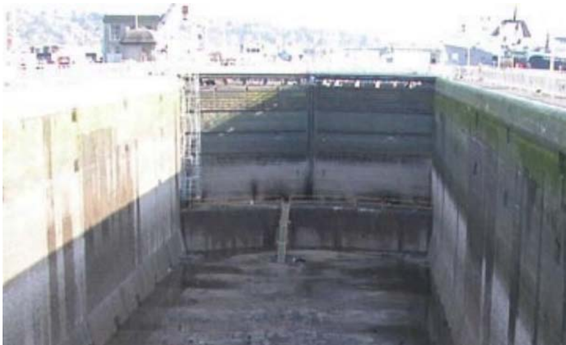
Figure 1.8 Photograph showing the cill and gates structure of a lock 18
