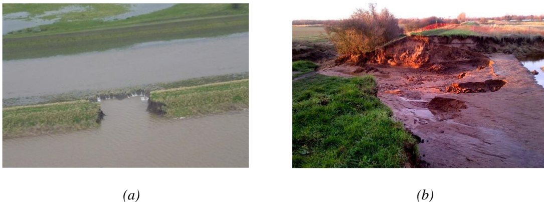
Figure 4-1: Examples of Breaches in riverine embankments. (a) Croston Breach Winter Floods 2015/2016, Lancashire (Simm et al., 2017); (b) Tetney Breach, Yorkshire, 5th December 2013 (Environment Agency, UK)
