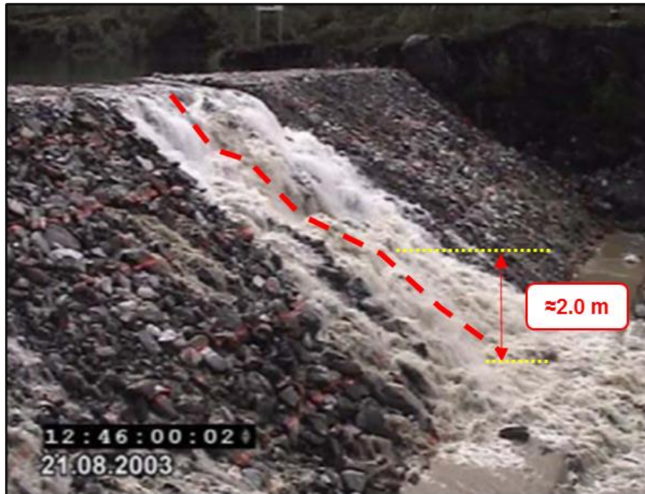
Figure 5-64: Interpretation of the IMPACT Field Test #3 embankment profile at the 46 minutes after the beginning of overflow
