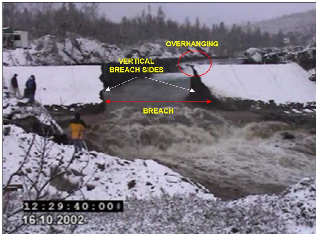
Figure 5-76: IMPACT Field Test #2 breach formation and growth, highlighting the vertical sides of the breach profile and overhanging material at the crest level.
