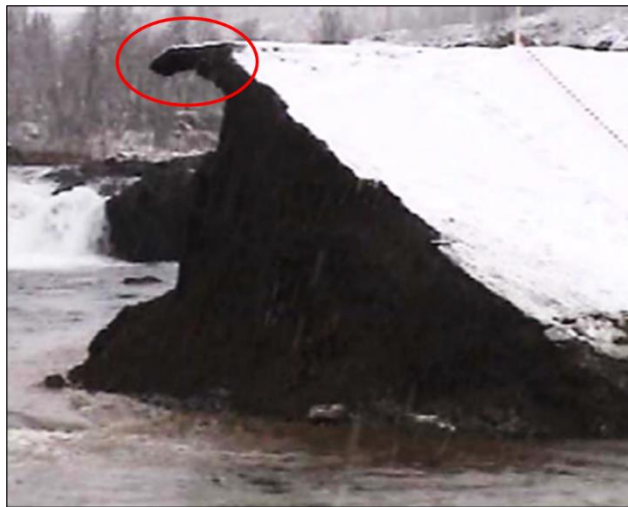
Figure 5-9: Breach side after test completion with overhanging region. (Morris, 2009)
