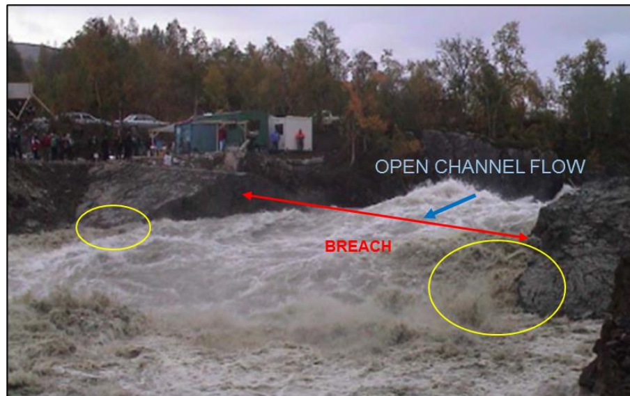
Figure 5-56: Final catastrophic failure showing the open channel flow through the breach
