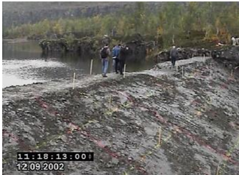
Figure 5-3: Homogeneous fine-grained test embankment (Impact, Test1-02)
