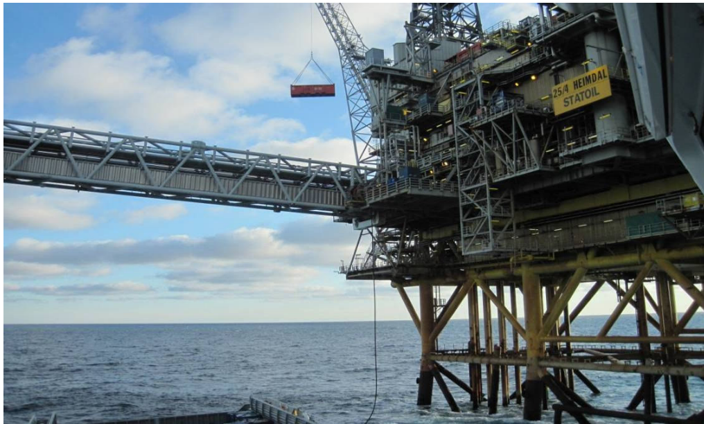
Figure 4.14: Offloading at Heimdal
