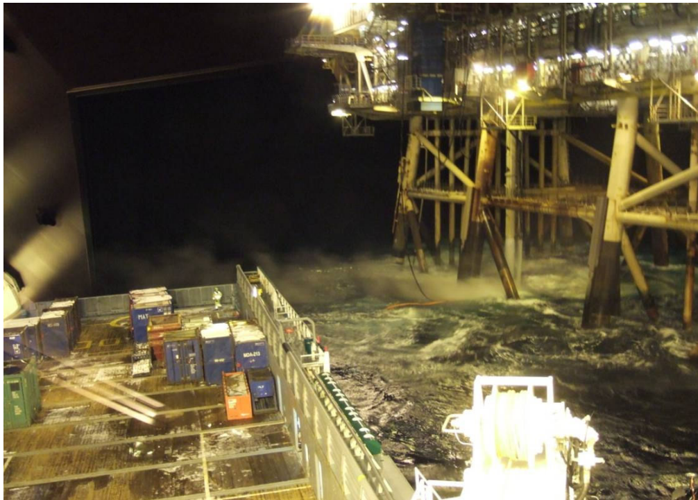
Figure 4.10: Night operation pumping liquids to and from tanks (hose in the water on port side of the vessel. To the right of the vessel in the photo.).
