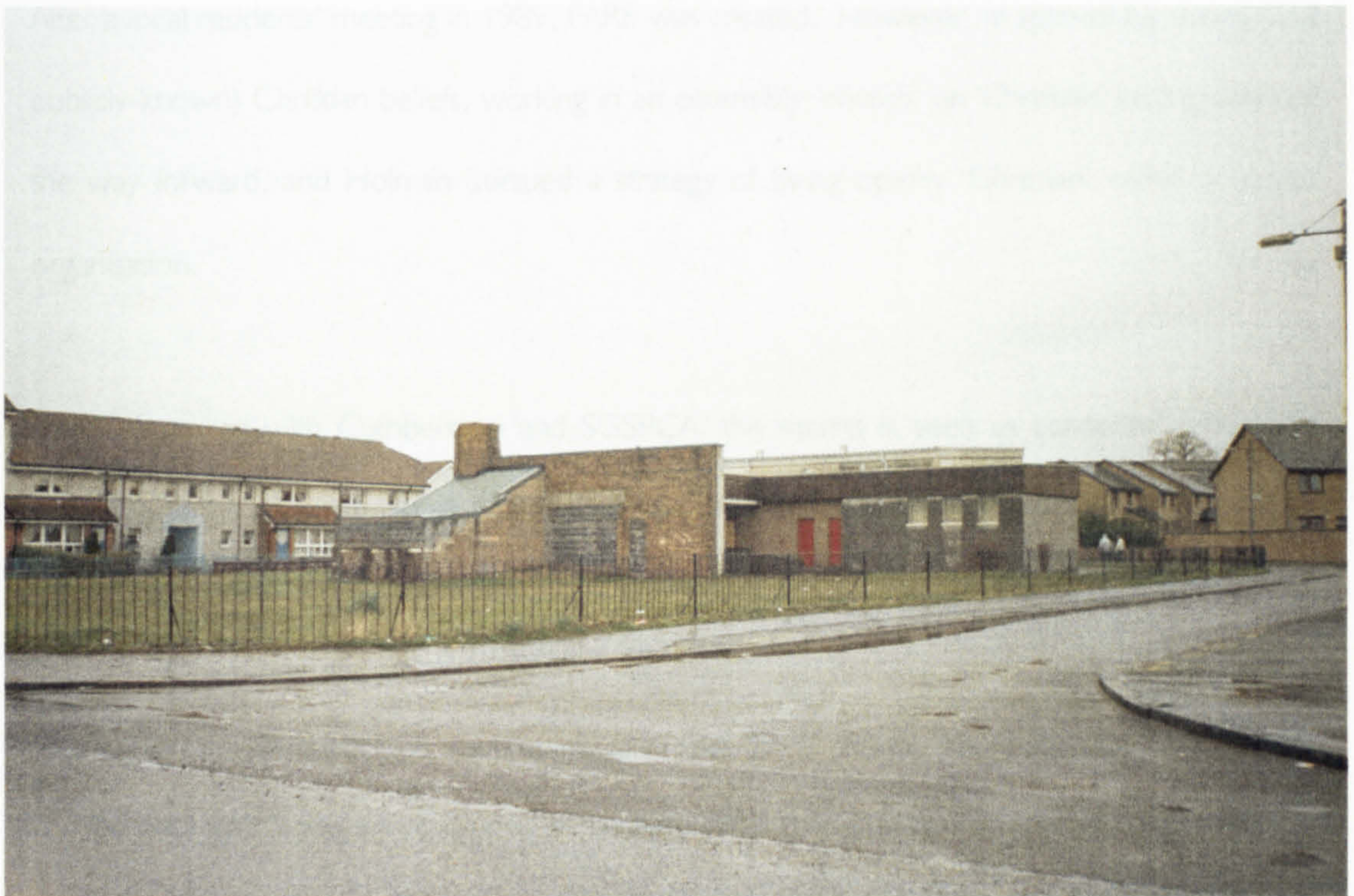
Plate 6.5 – Religious iconography in Easterhouse: St. George's & St. Peter's Church of Scotland, showing land in foreground where original sanctuary building was demolished due to lack of money for maintenance.
