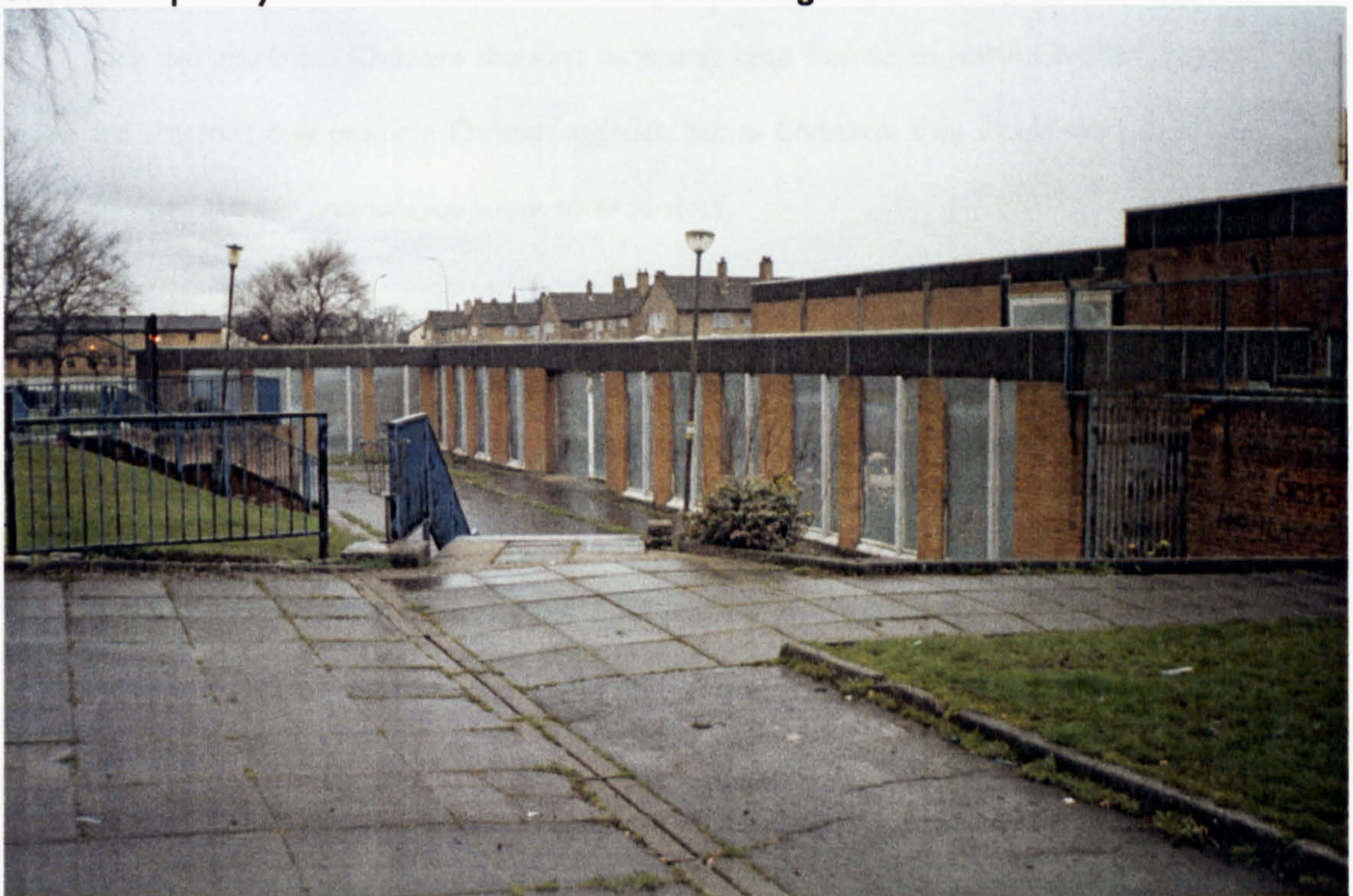
Plate 6.6 – Uninhabitable Easterhouse: boarded-up tenements and the former community centre occupied by SGSPCA before withdrawal of funding.
