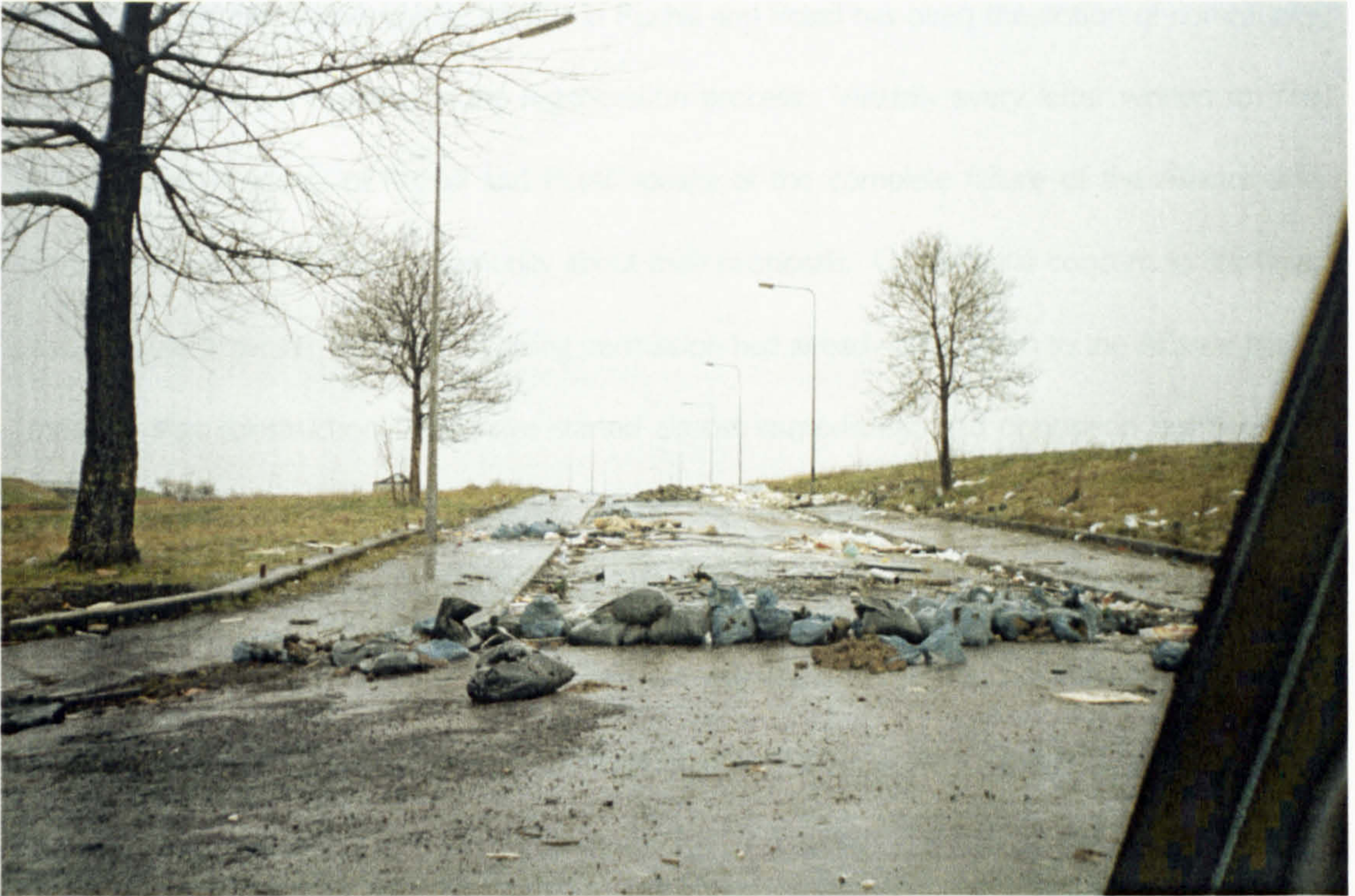
Plate 6.7 – The ‘Glasgow Lowland Clearances’: Possilpark, following wholesale demolition of local authority tenement housing.
