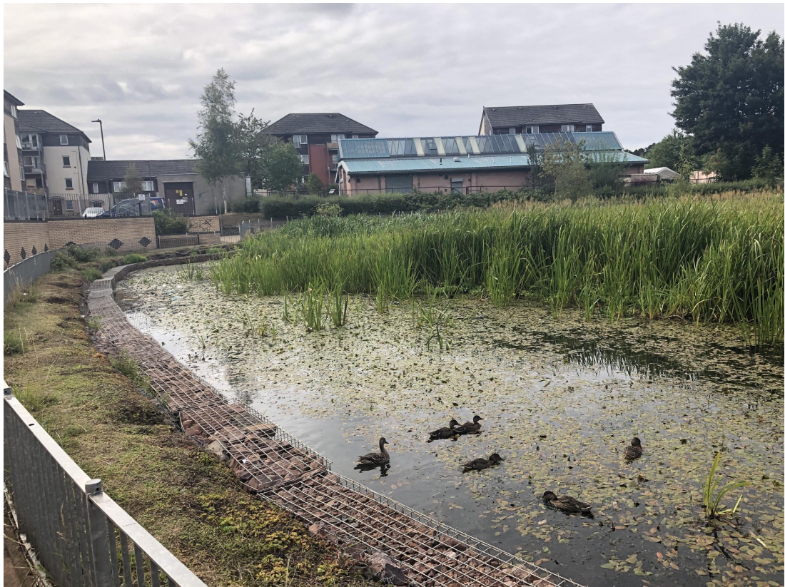
Figure 1.3: Retention pond in Edinburgh, Scotland.
