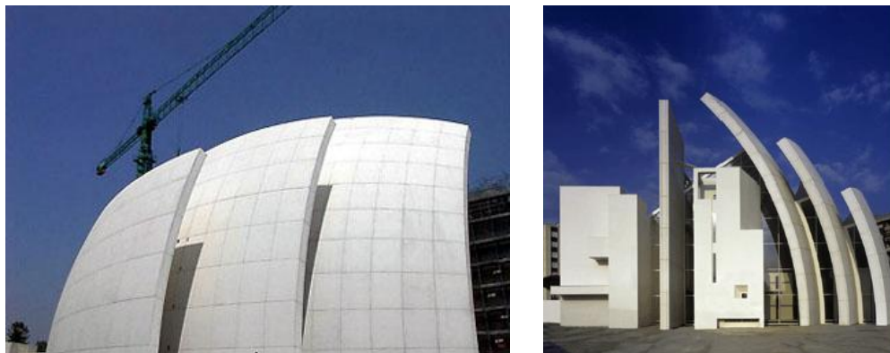
Figure 1-10 the Jubilee church in Rome features an anti-staining titania coating 27
