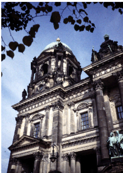
Figure 3-1 Airborne soot particles discolour stonework as well as causing health problems 1
