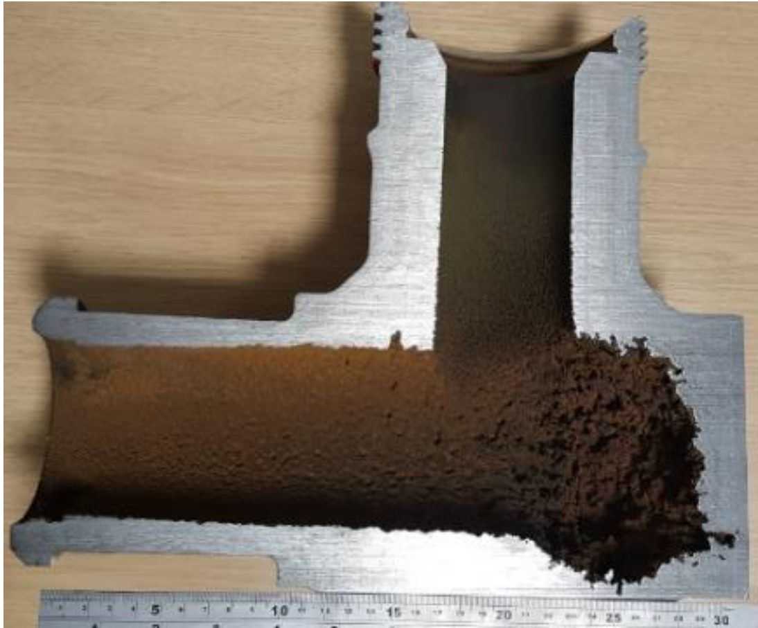
Figure 1.2: 90° elbow which has suffered severely from erosion-corrosion damage (courtesy of WSPM)
