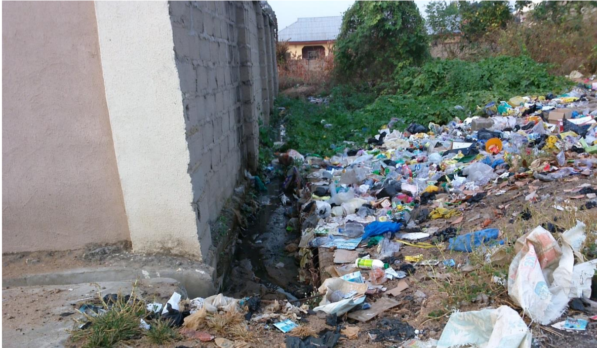
Figure 4.2: Refuse dump on private property/ drains blockage
