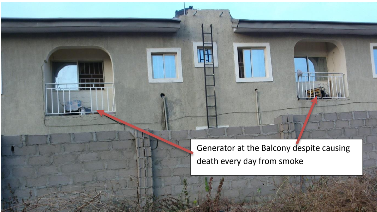
Figure 4.5: Conversion of balcony to generator house
