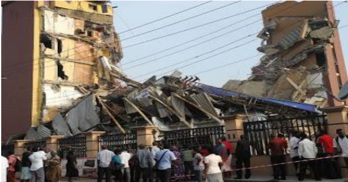
Figure 3.5: Catastrophic Structural MRRB Failure
