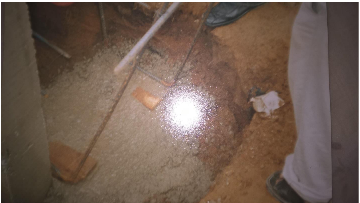
We met this group placing staircase starter, no professional except an elderly brick layer in charge of the work
