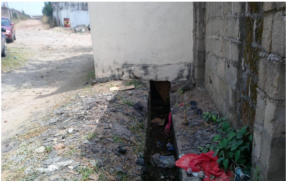
Figure 4.7 Access road/drainage blocking and conversion to personal property
