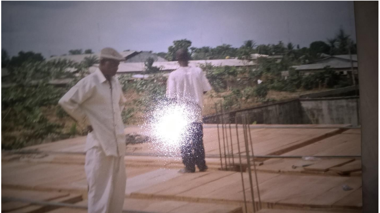
A brick layer supervising first floor reinforcement placements
