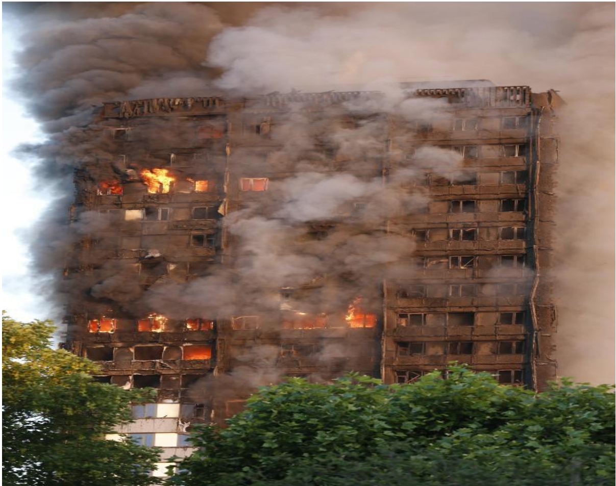
Figure2.6 Grenfell fire safety regulation violations (Source: Google earth)
