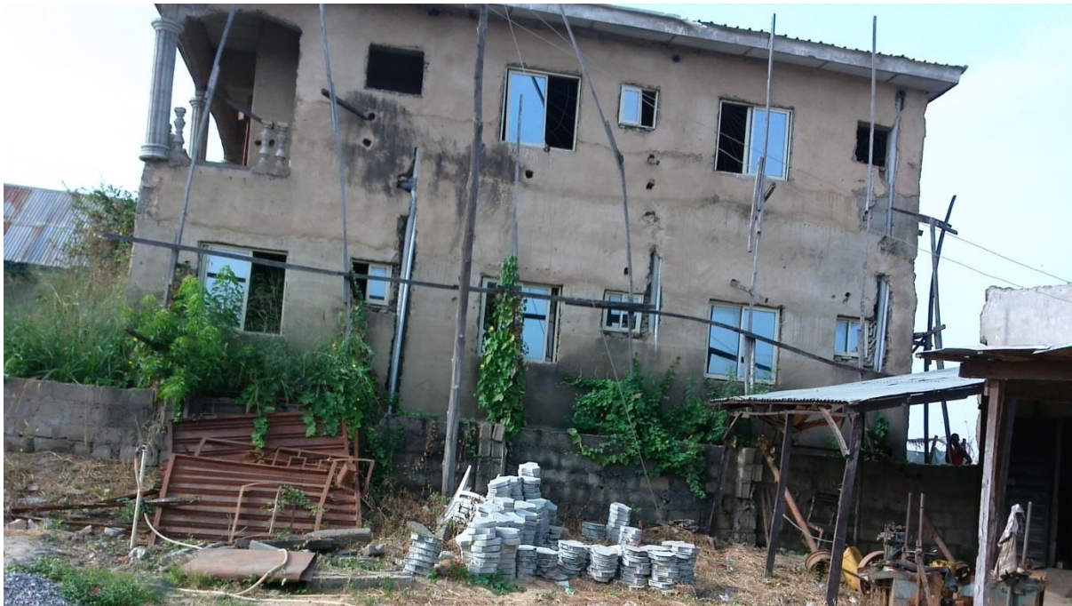
Figure 4.4: Sub-standard housing building construction
