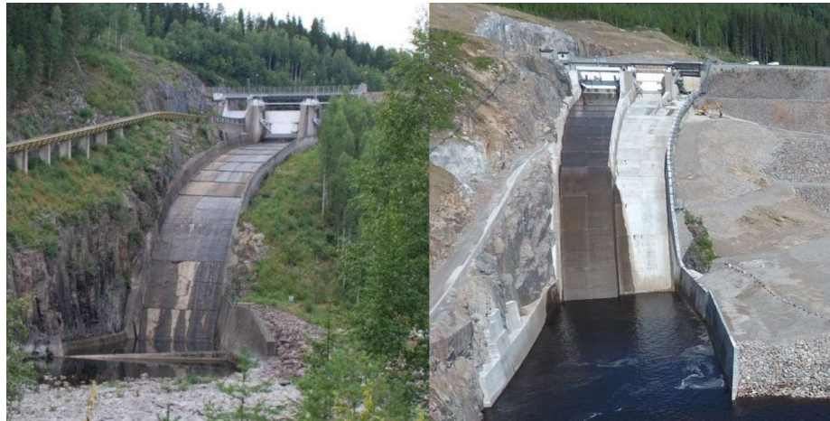
Figure 1.1: The spillway of the Höljes dam (Sweden) with the original layout with two gate openings (left) and after refurbishment with a new 17 m gate opened next to the existing gates to accommodate increased discharge (right). Reproduced with permission, Copyright 2019, Yang et al. [22].
