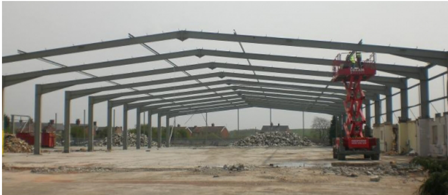
Figure 3.1: Typical portal frame building
