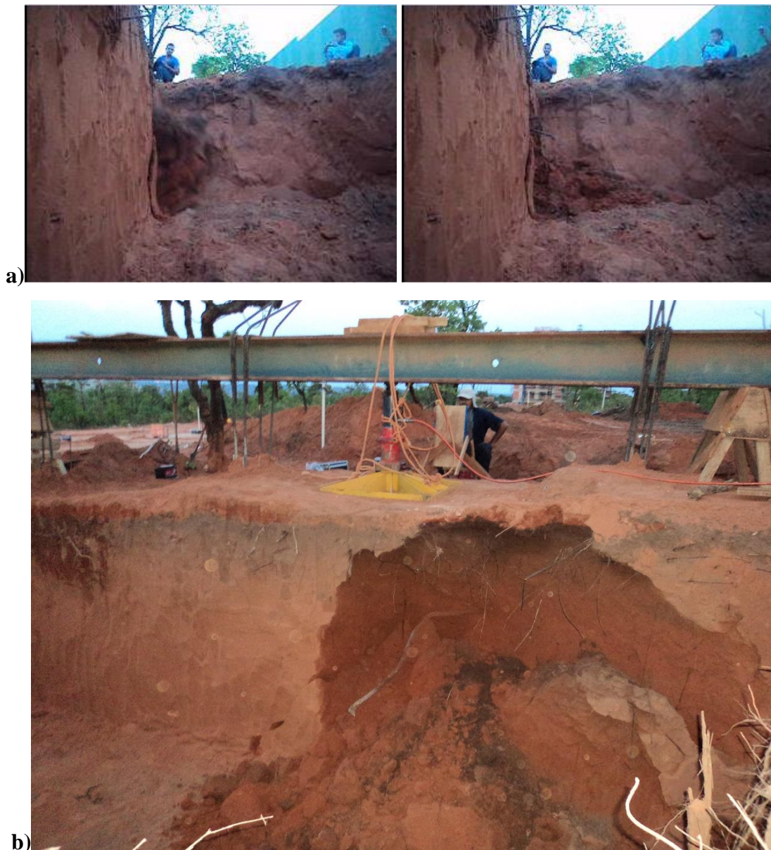
Figure 8.14: The FT2 No1 failure event (FT2: soil block topple and fall), Experiment L1. After cracks surrounded a volume of soil, it was detached from the vertical face of the landslide. The FT2 No2 involved a) soil blocks toppling and b) falling on ground surface and was the most complex one observed in both landslide experiments. FT2 No1 was one of the two largest failure events that occurred during both Experiments L1 & L2.
