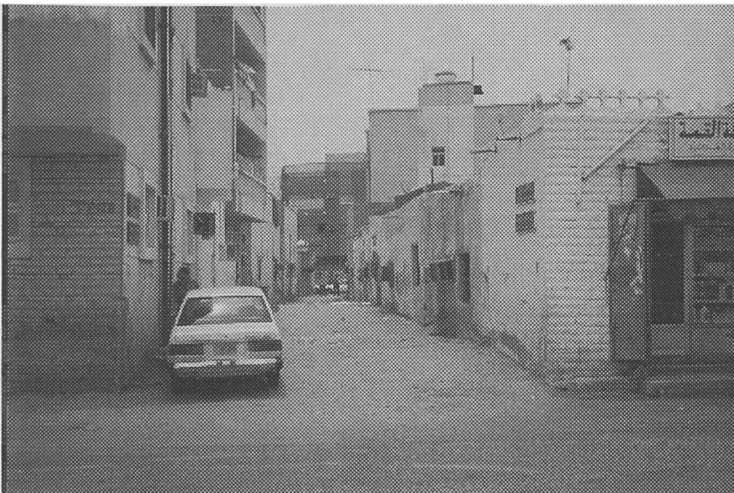
Figure 2.6 Madain Al Fahad District. Low socio-economic district located in the old sector of Jeddah City. View along passageway, but wider than in Fig. 4.9. Paved surface. No pavements. Small supermarket on right of picture. Buildings 2 or 3 storeys. Most houses have air conditioning units.
