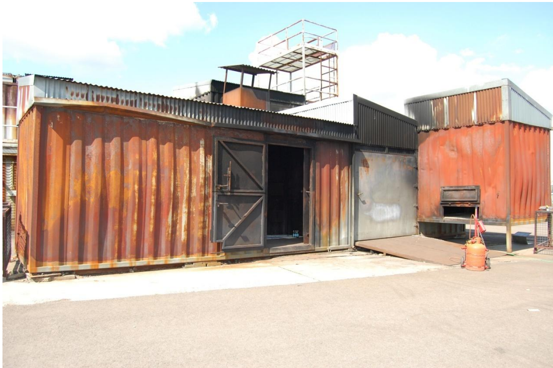
Figure 5-1 Image of Grampian Fire and Rescue training facility
