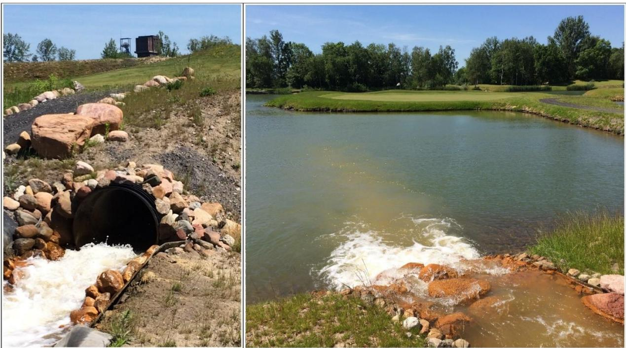
Figure 2.6 The pumped mine water discharge from Ewa shaft in Bytom, Poland (left), and its outfall into a lake within the ARMADA housing development complex (right). Photos reproduced with permission of © David Banks
