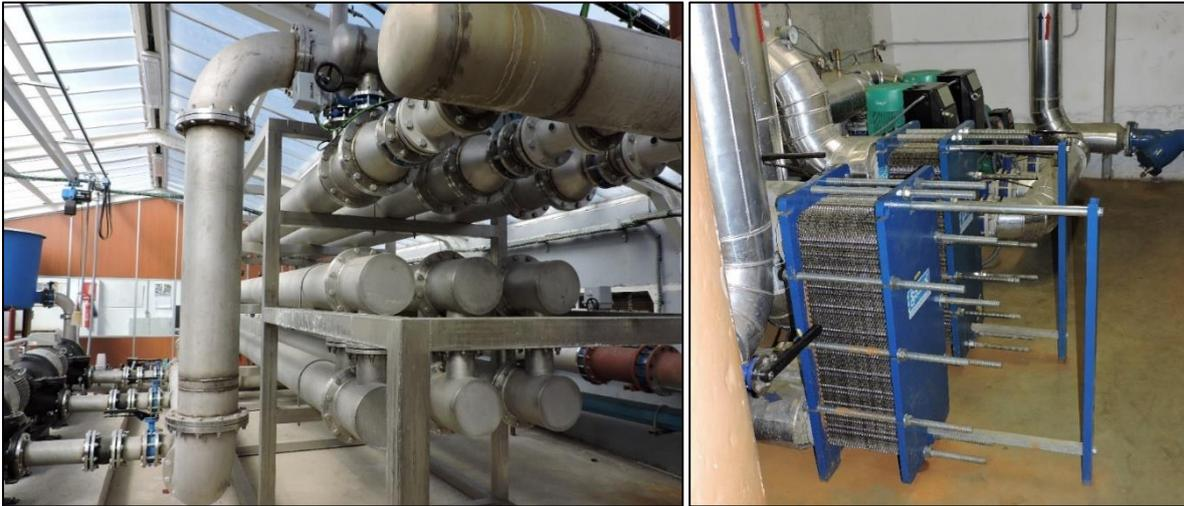
Figure 2.5 (left) Shell-and-tube heat exchangers between minewater and secondary circuit to hospital, Barredo shaft-top building; (right) minewater to secondary circuit plate heat exchangers. University plant room. Photos by © David Banks.
