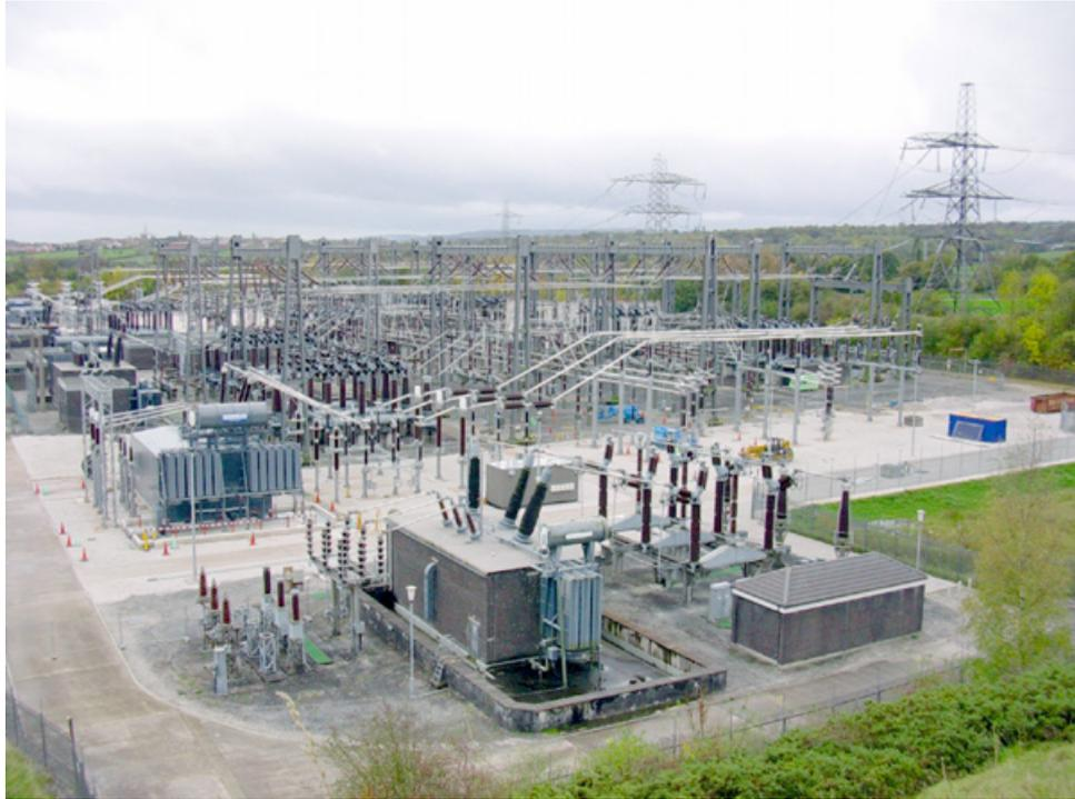
Figure 2.1: An example of an air-insulated substation. National Grid Legacy station nr. Wrexham, Wales
