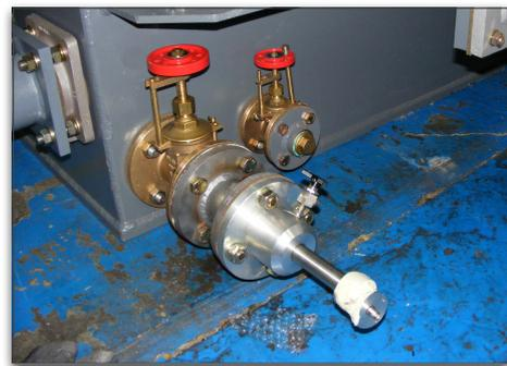
(b) An example of a UHF probe sensor mounted on a gate valve
