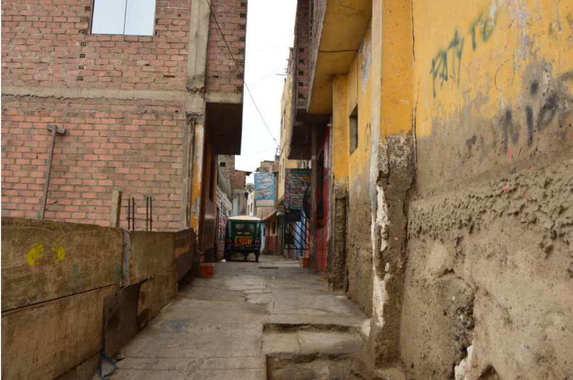
Figure A.38: San Pedro. Pedestrian street
