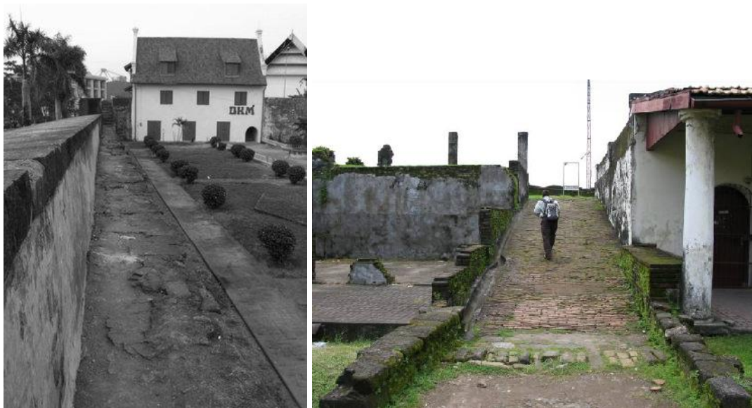
Figure 2.63 The passageway, 2008 (Source: NTQT, Malaysia)
