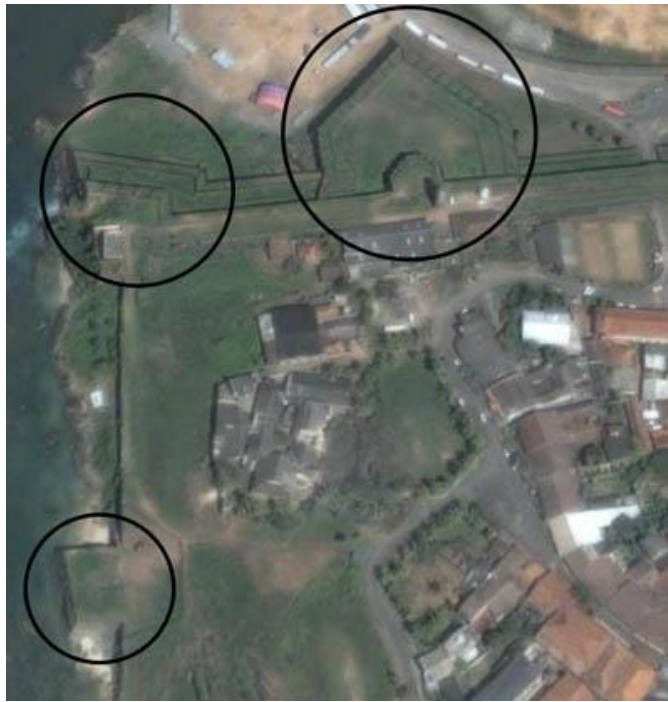
Figure 2.6 Various types of bastions at the Galle fortress, Sri Lanka, 2009 (Source: Google Earth)
