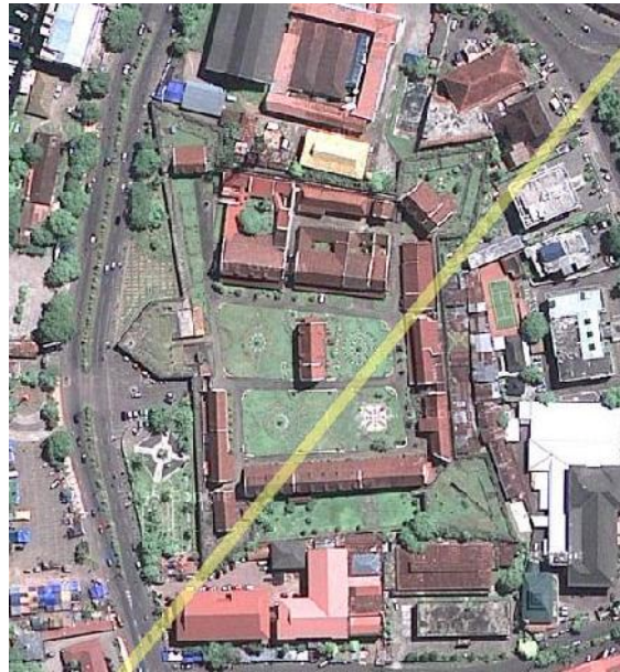
Figure 2.56 Location map(top) and satellite view of Rotterdam fortress(below), Makassar, 2009 (Source: Google Earth)
