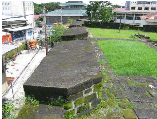
Figure 2.65 Crenel at the bastion of Rotterdam fortress, 2008 (Source: NTQT, Malaysia)
