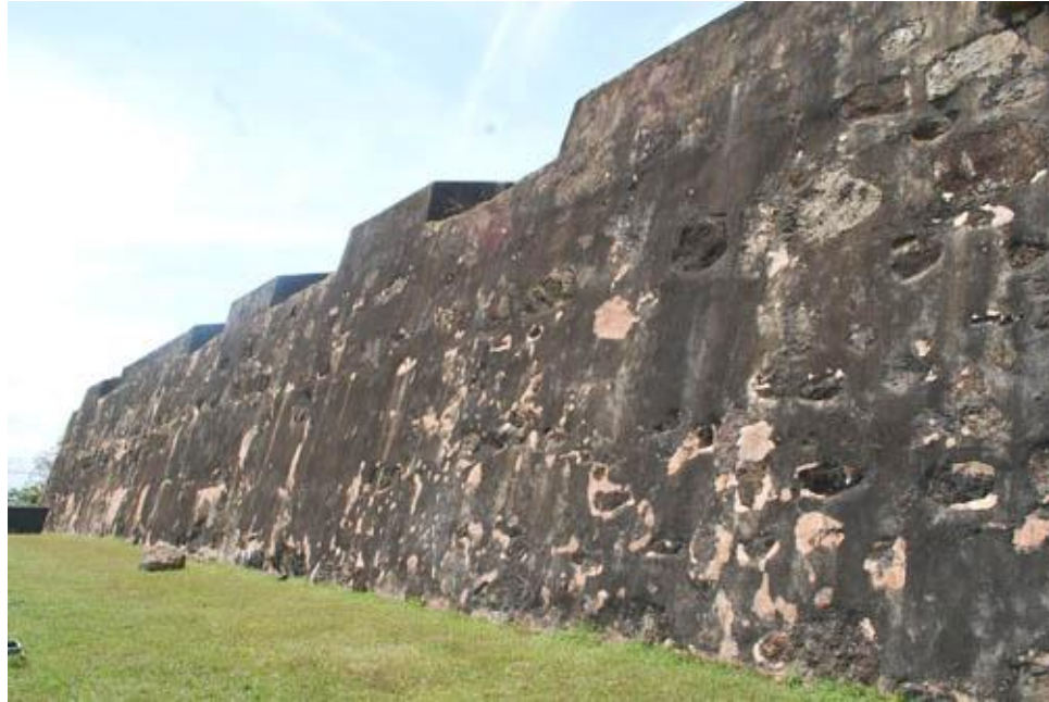
Figure 2.44 Solid granite stone as the main material of Galle fortress, 2009 (Source: Author)
