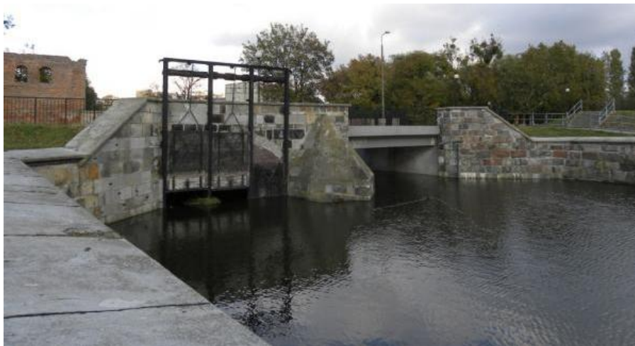
Figure 2.18 Example of the stone sluice (Source: http://www.penninewaterways.co.uk )
