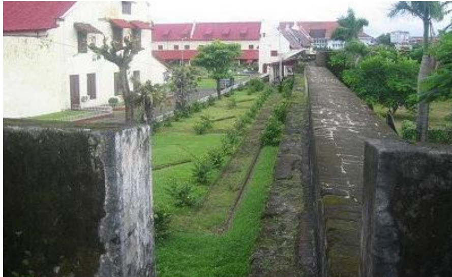
Figure 2.64 The parapet, 2008 (Source: NTQT, Malaysia)
