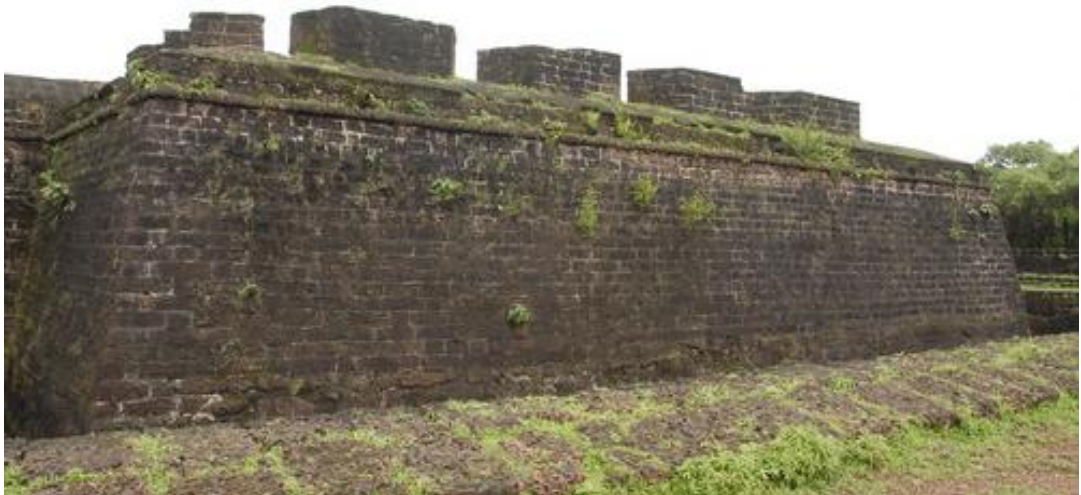
Figure 2.37 Crenels at one of the bastions, 2009 (Source: Author)
