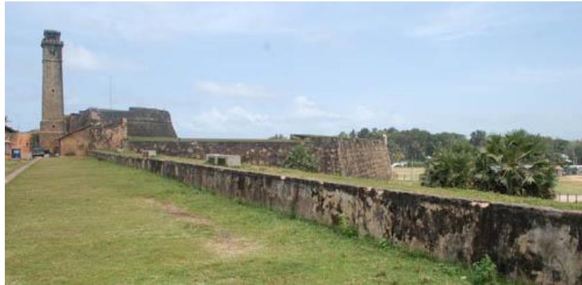
Figure 3.46 Bastion wall is normally higher than other walls, Galle fortress (Source: Author)
