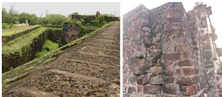
Figure 2.31 The use of laterite as main material in both fortresses, Aguada fortress (left) and Porta de Santiago gate of the A Famosa fortress, 2009 (right) (Source: Author)
