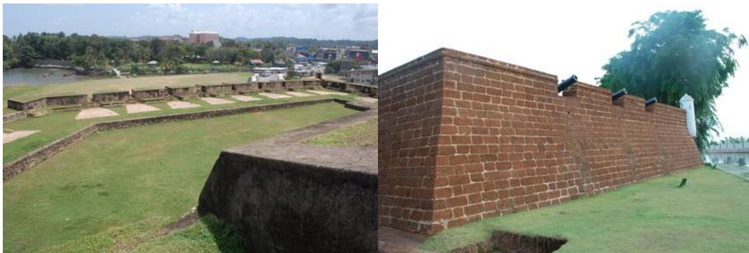
Figure 2.50 Crenel at the Galle fortress (left) and the reconstruction at A Famosa fortress (right), 2009 (Source: Author)
