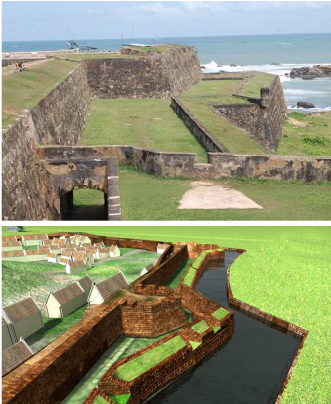
Figure 4.35 Fausse-braie at Galle fort in Sri Lanka (above) being used as a reference for modelling Fausse-braie at A Famosa fort (below)(Source: Author)
