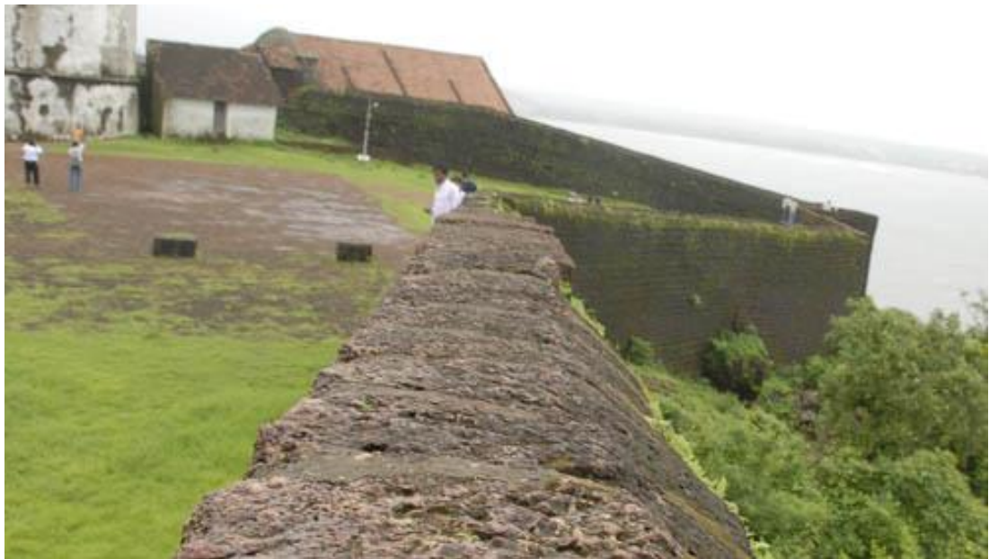
Figure 2.36 The parapet that encircles the fortress, 2009 (Source: Author)
