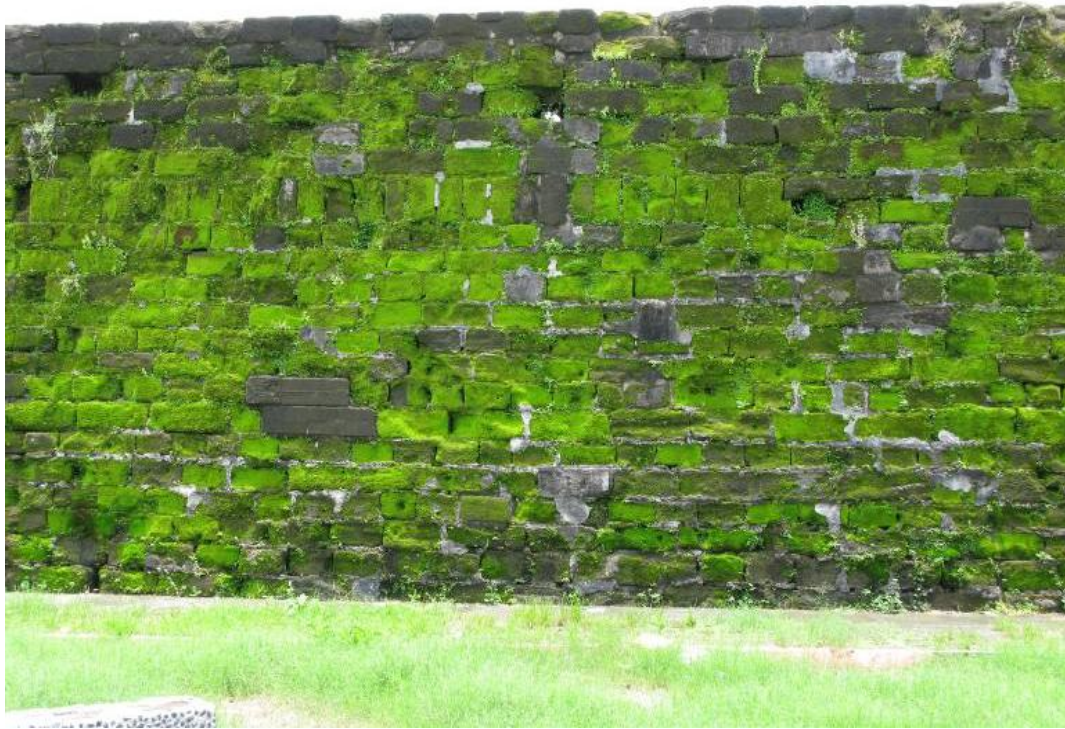
Figure 2.60 Brick and limestone as the fortress's material, 2008 (Source: NTQT, Malaysia)
