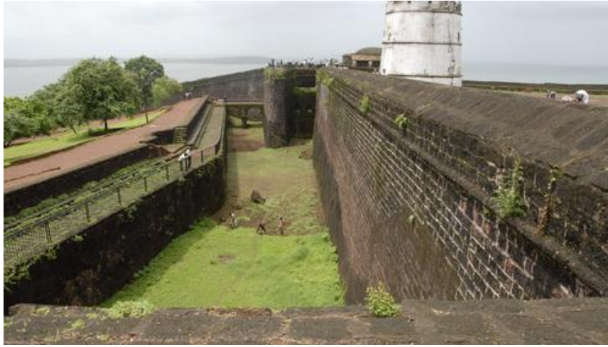
Figure 2.4 Artificial fortification: Fort of Aguada, 2009 (Source: Author)
