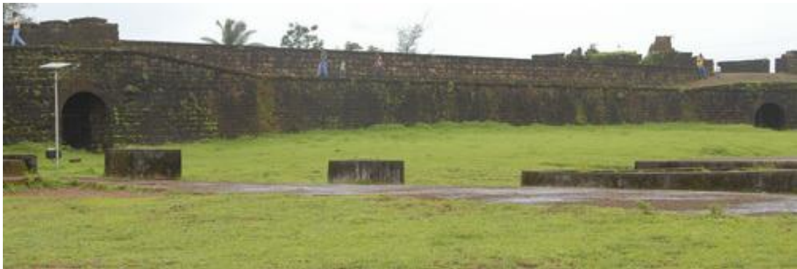
Figure 2.34 Passageway of the fortress, 2009 (Source: Author)
