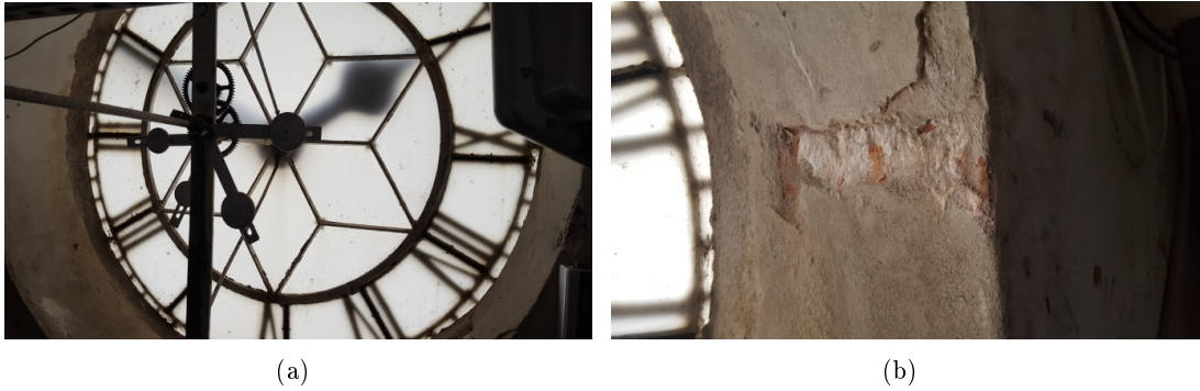
Figure 5.3: Image of the clock window from inside the Clock Tower, Lerwick Town Hall (a) and detail of the deteriorated surrounding, showing the outer render and underlying brick work, Lerwick Town Hall (b).
