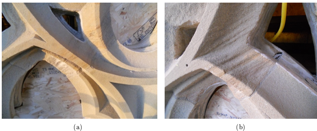
Figure 5.8: Images of bedding planes: area of sampling of SM1, at the top of the left side of the right window (from outside) on the south side of the main hall, first floor (a) and magnification of another bedding plane on the right side of the left window.
