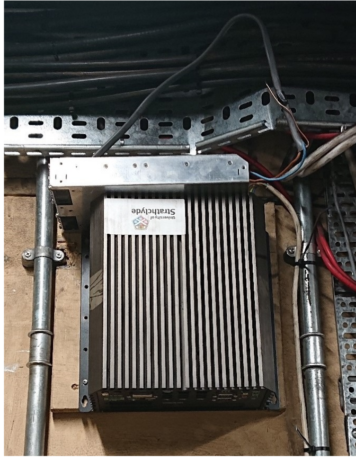
Figure 6.22: Installation of the 5GRN BBU in the SPT Communications Room.
