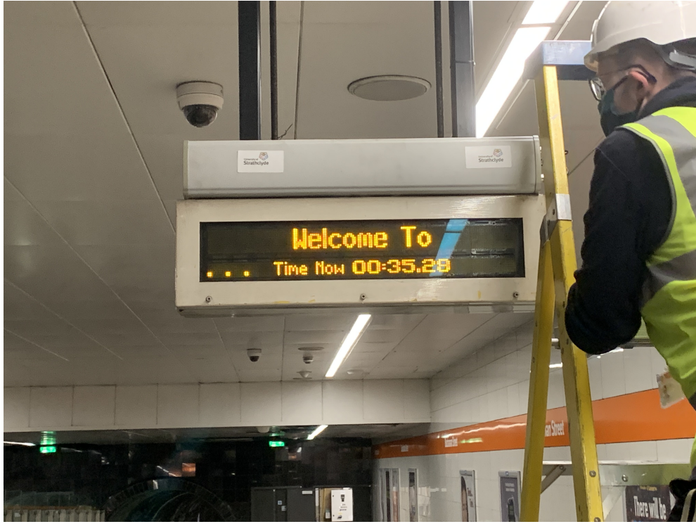
Figure 6.21: The author installing the AW3014 directional antenna at Buchanan Street Subway Station.
