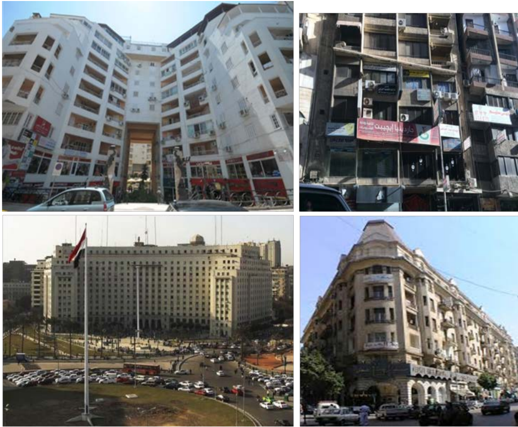
Figure 3-3. Examples of the third category of Egyptian commercial buildings - whole or part of existing buildings.
