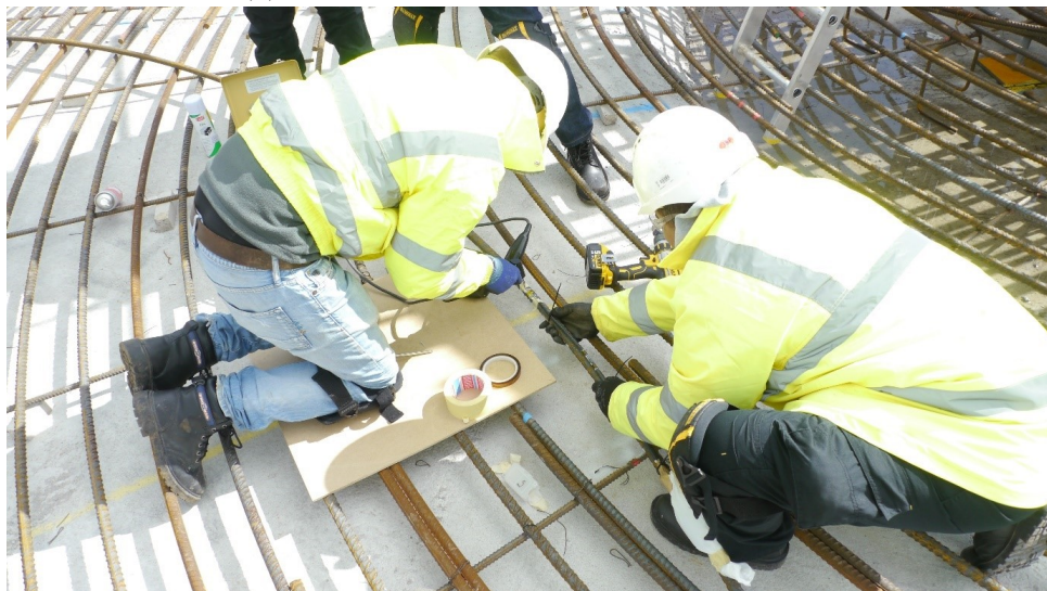
(b) Sensor installation inside of the foundation
