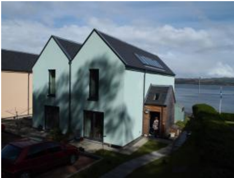
Figure 6.17 - Dunoon PassiveHouse – Note Solar Thermal Panel Installation
