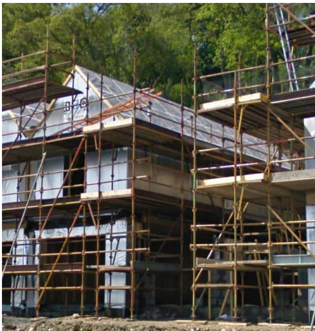
Figure 6.19 – Energy Efficient Home during build, part of the Tigh-Na-Cladach development
