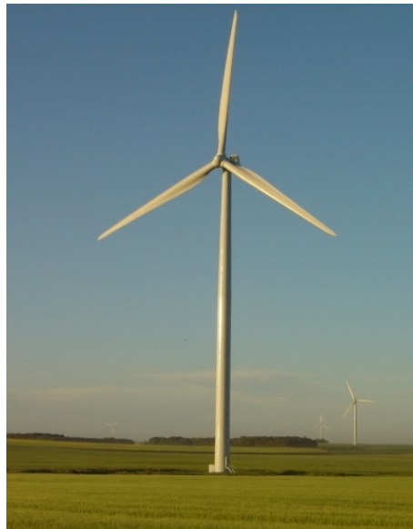
Figure 2.1: A typical modern 3 bladed wind turbine
