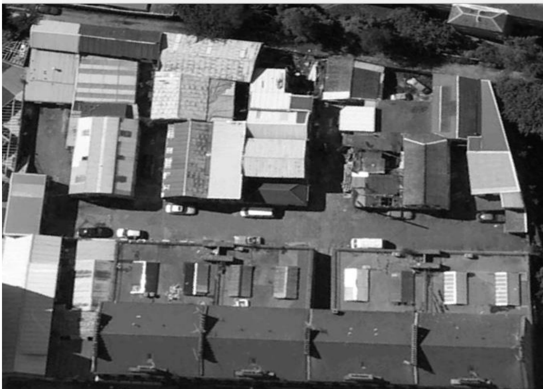
Figure 8: Aerial Shot of Argyle Court
