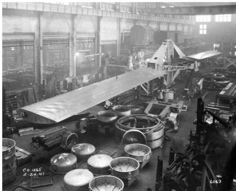
Figure 2.2: Construction of the Smith-Putnam Wind Turbine [13]
