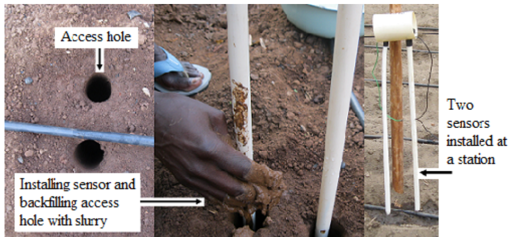
Fig. 4.9: Installation of sensors in the field
