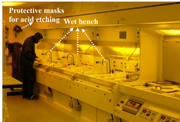
Figure 2-10: Photograph of the wet bench in our cleanroom.
