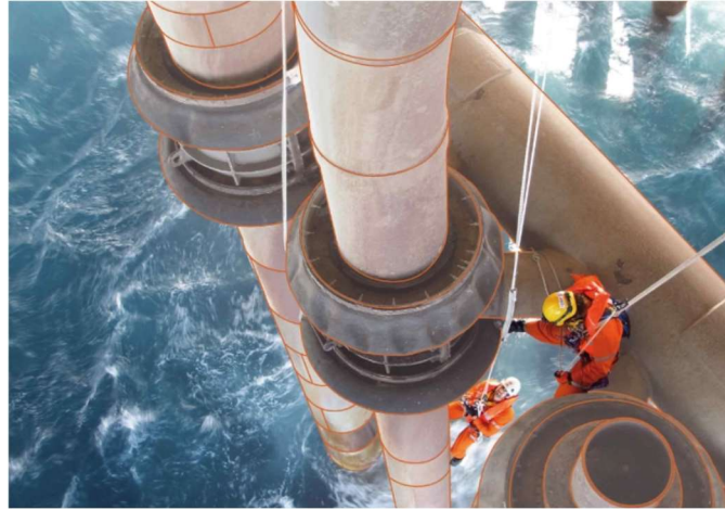
Figure 1-2: Example of work at height conducted from an offshore platform [18].
