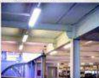
This LED light fitting has been manufactured from corrosion resistant glass reinforced polyester and contains a
