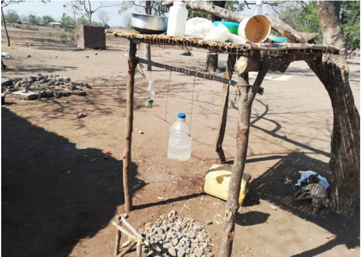
Figure 30: Tippy Tap handwashing facility under a dish rack
