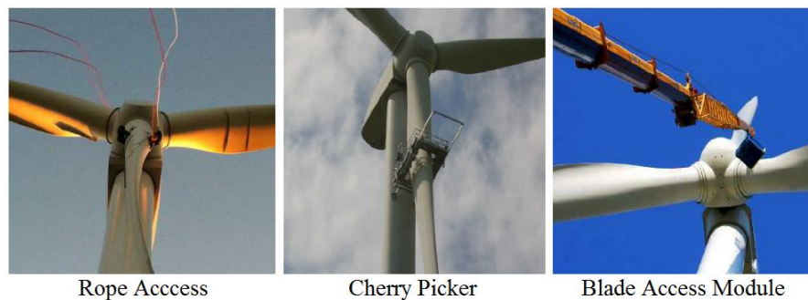
Figure 3-10. Blade access techniques. Source: [88]
