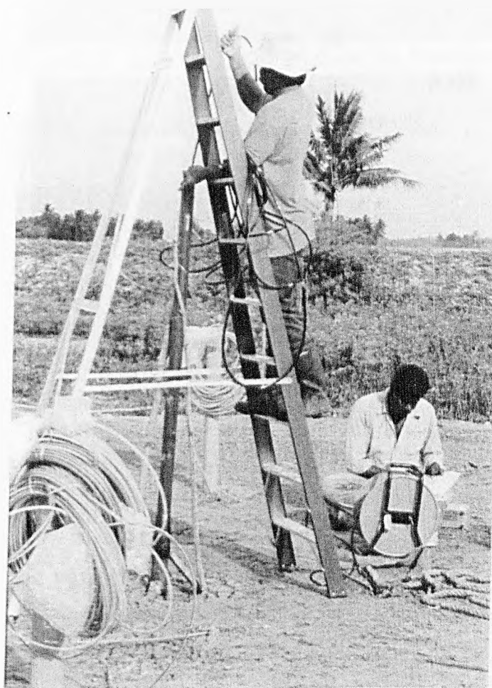
Plate 4.12 : Insertion of Torpedo Probe to Take Readings of the Inclinometer
