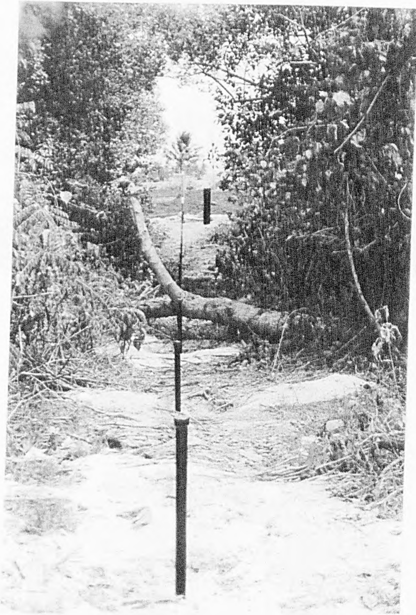
Plate 4.17 : Heave Markers Installed Near the South Trial Embankment
