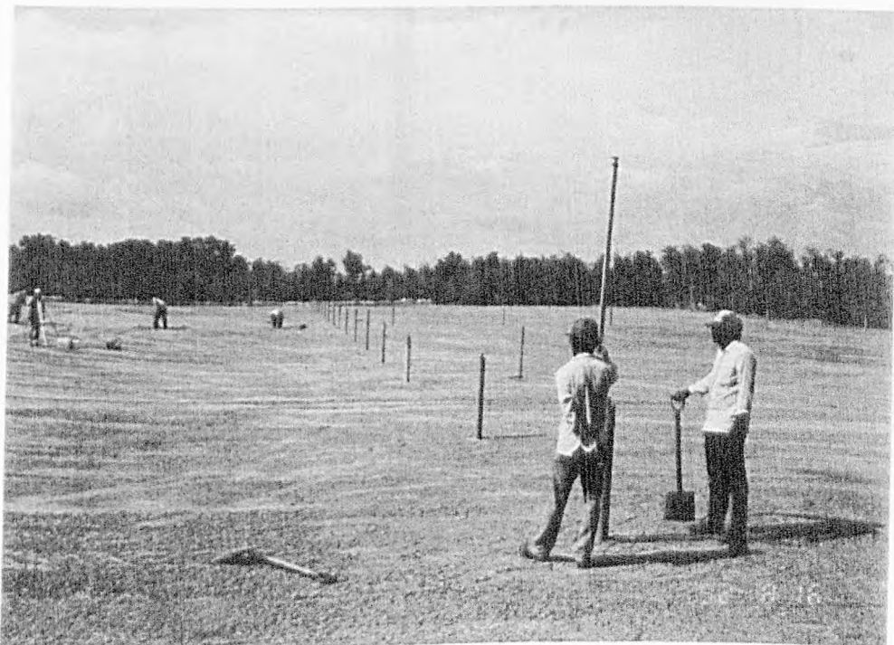
Plate 4.16 : Taking of Reduced Levels of Settlement Plates
