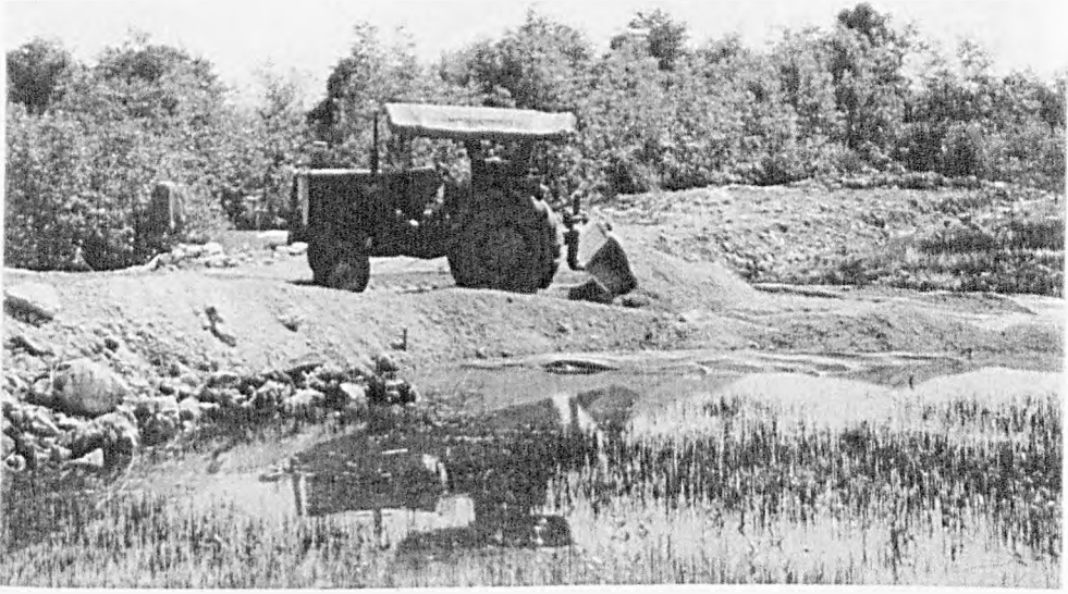
Plate 4.5 : Levelling of the Drainage Material by Backpushers
