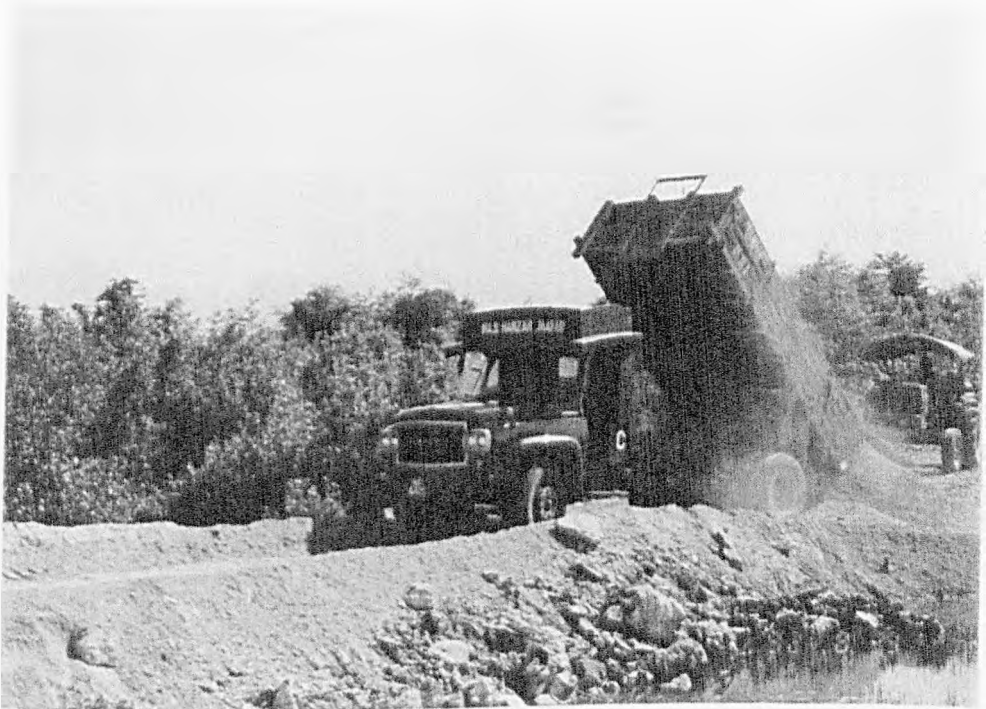
Plate 4.4 : Dumping of Drainage Material by Lorries
