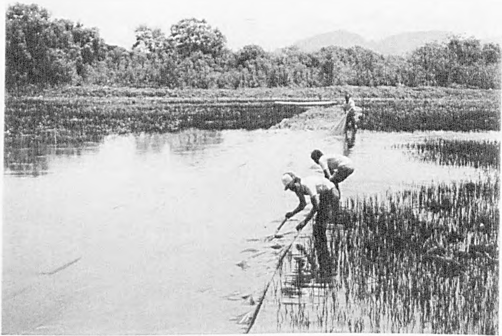
Plate 4.3 : Pegging the Geotextile by Wooden Stakes
