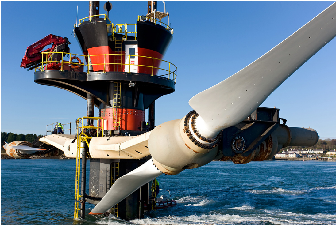
(a) MCT SeaGen dual 600 kW turbines at Strangford Lough, Northern Ireland, UK (Siemens press picture, copyright Siemens AG, Munich/Berlin)
