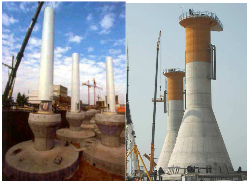
Figure 1.9. Shallow water (to the left) and deep water (to the right) gravity based foundations [14]
