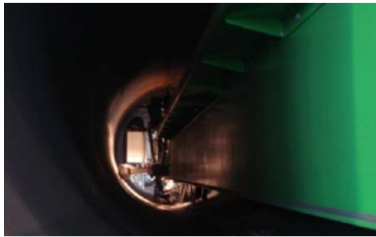
Figure 3.18. Monopile manufacturing. Inside circular welding [82]
