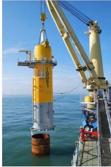
Figure 3.27. Transition Piece being placed above driven pile [87]
