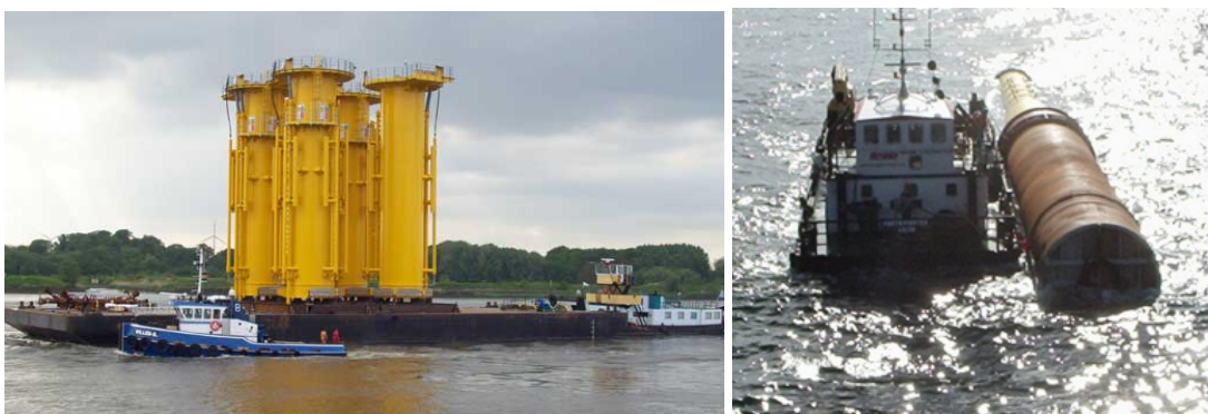
Figure 3.32. TP transportation by barge [96] and flotation [85]
