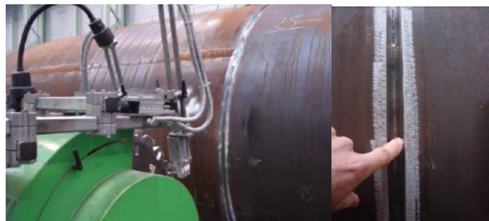
Figure 3.19. Monopile manufacturing. Milling of the circular union [82]
