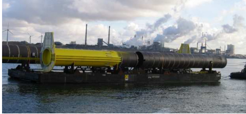
Figure 3.25. Whole monopile structure (pile+TP) transportation in one piece [85]
