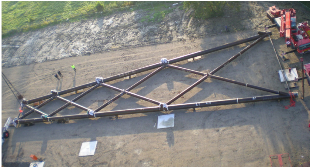
Figure 3.36: Assembled part of jacket substructure [46]
