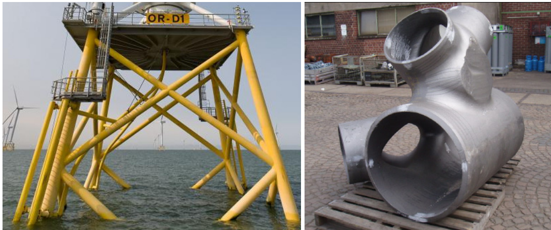
Figure 3.35: Welded joints [104] (to the left) and cast node [46] (to the right) comparison
