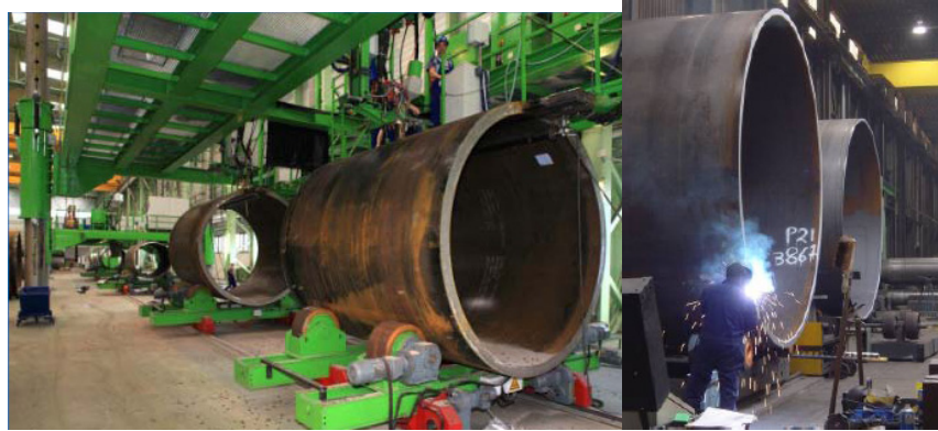
Figure 3.15. Monopile manufacturing. Outside longitudinal welding [82]
