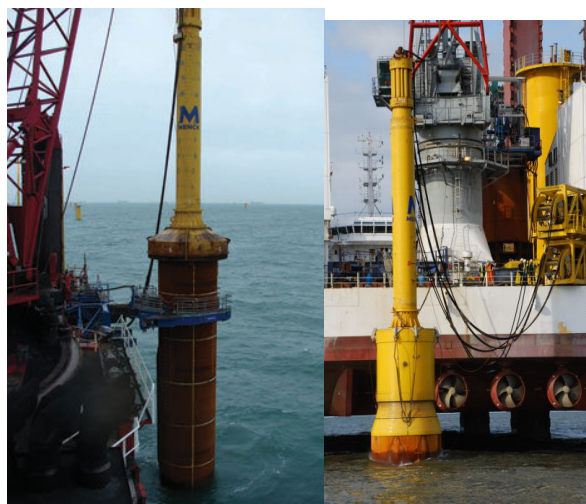
Figure 3.24. Offshore pile driving [14]
