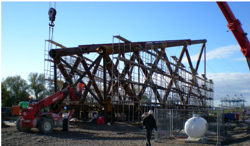
Figure 3.37: Erection of a jacket substructure [46]
