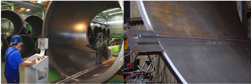
Figure 3.13. Monopile manufacturing. Inside longitudinal welding [82]
