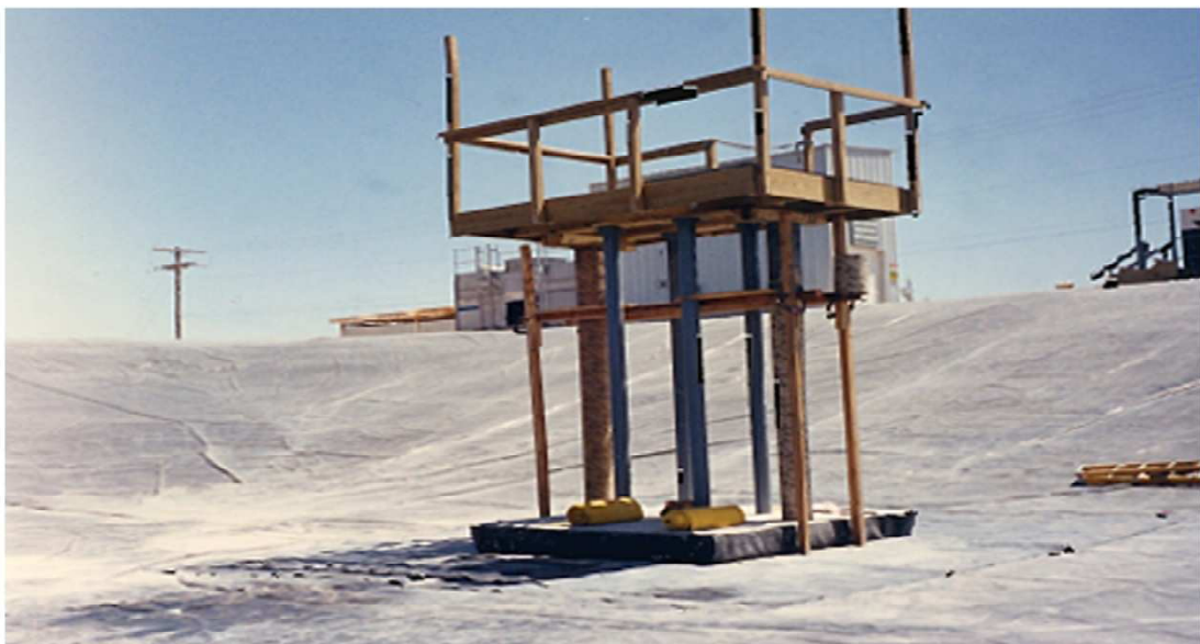
FIGURE 2.14. Instrumentation tower shown in yellow in the middle of the pond [26].
