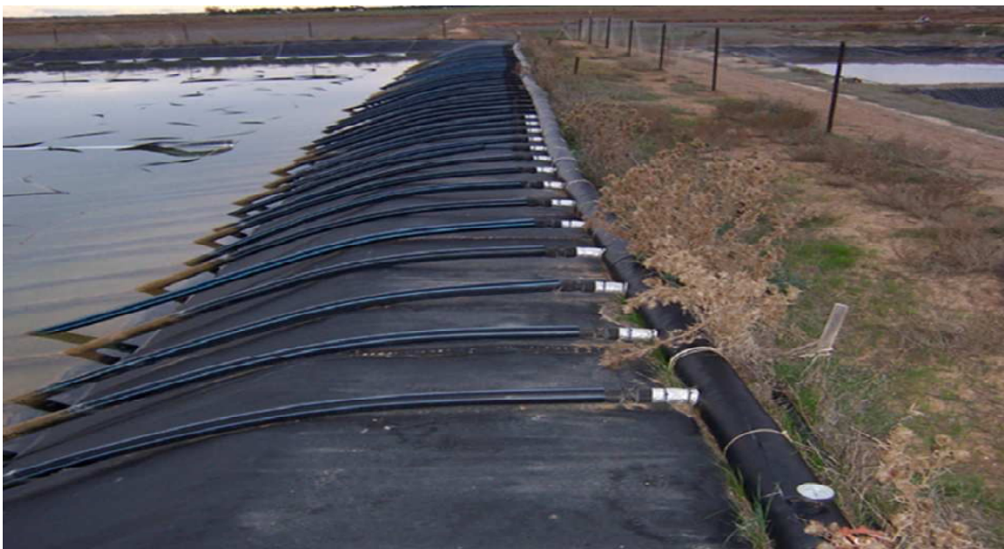
FIGURE 2.19. Heat extraction tubes and inlet manifold at Pyramid Hill [26].
