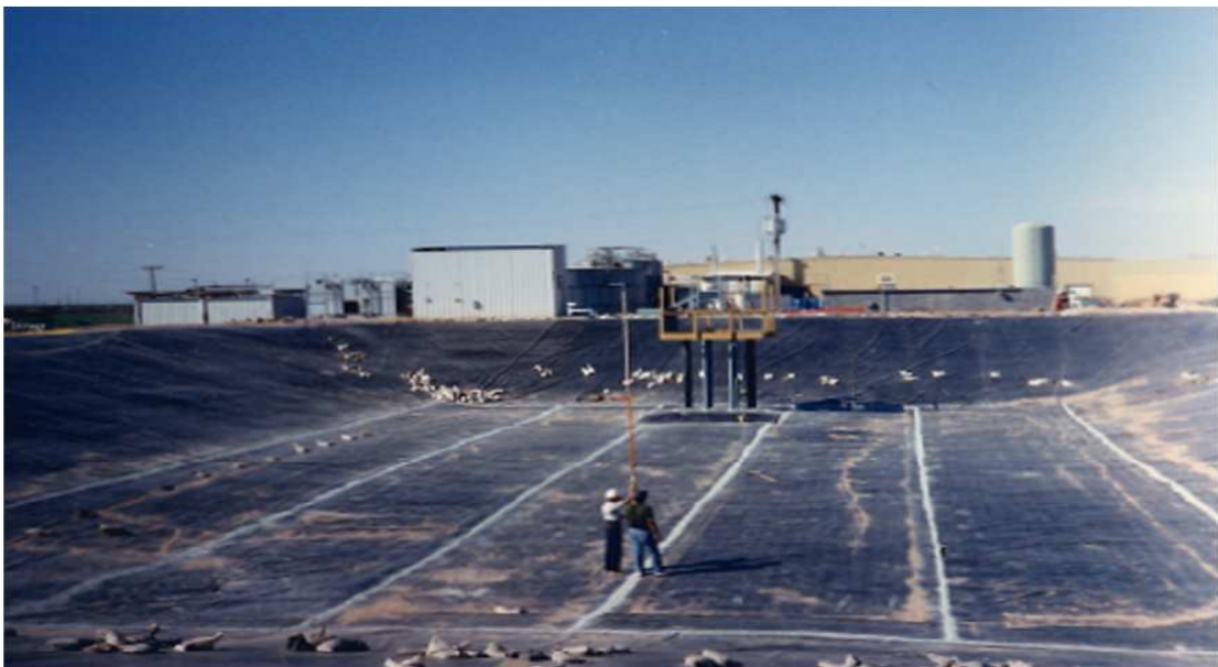
FIGURE 2.9. SGSP with liner system installed at El Paso [25].
