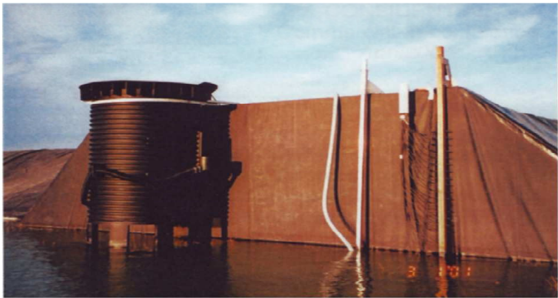
FIGURE 2.13. Salt charger fixed to interface wall [26].
