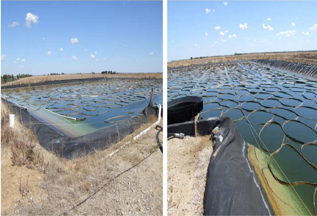
FIGURE 2.5. Pyramid Hill solar pond, Australia. The floating rings shown are wind suppressors to minimize the wind effect [26].
