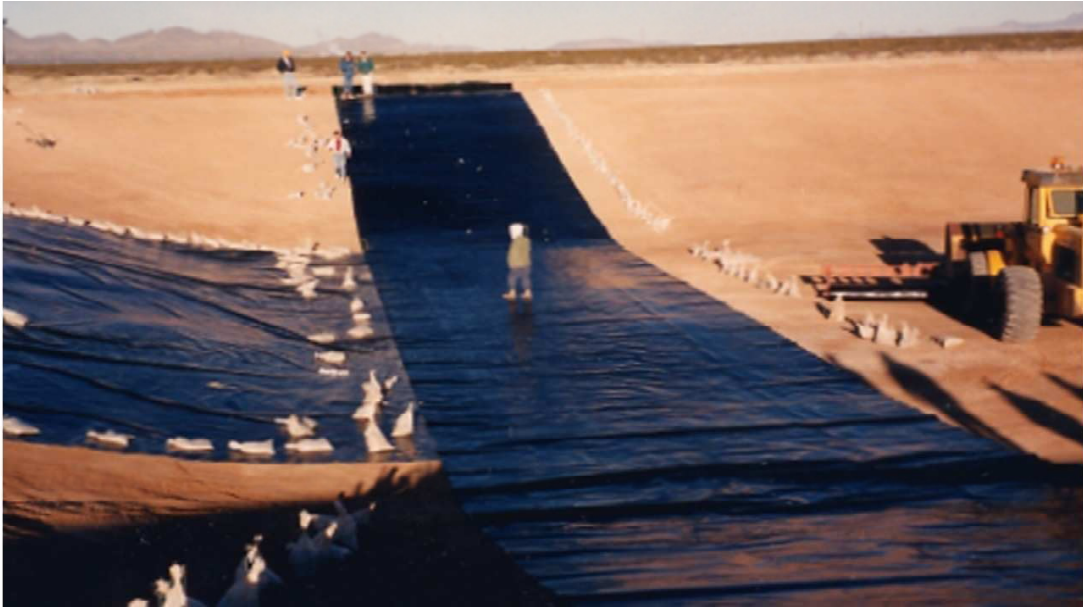
FIGURE 2.8. Installation of the flexible polypropylene geomembrane liner [25].
