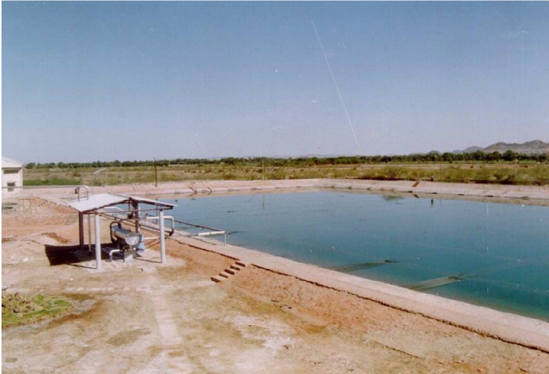
FIGURE 2.4. Bhuj solar pond, India [33].
