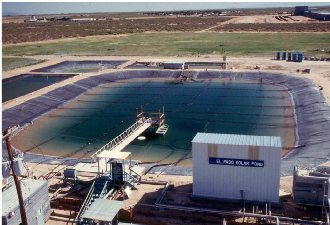
FIGURE 2.3. The El-Paso salinity gradient solar pond [26].
