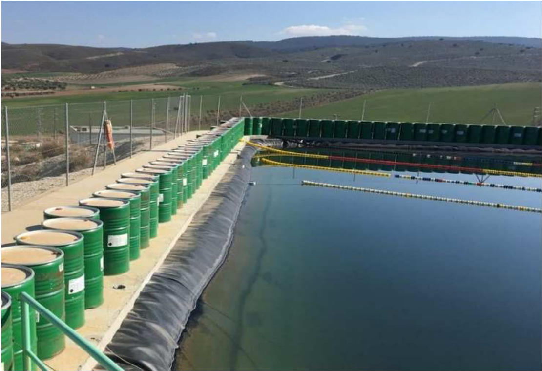
FIGURE 2.6. Granada industrial solar pond, Spain. The barrels role is to protect the pond from the wind [27].
