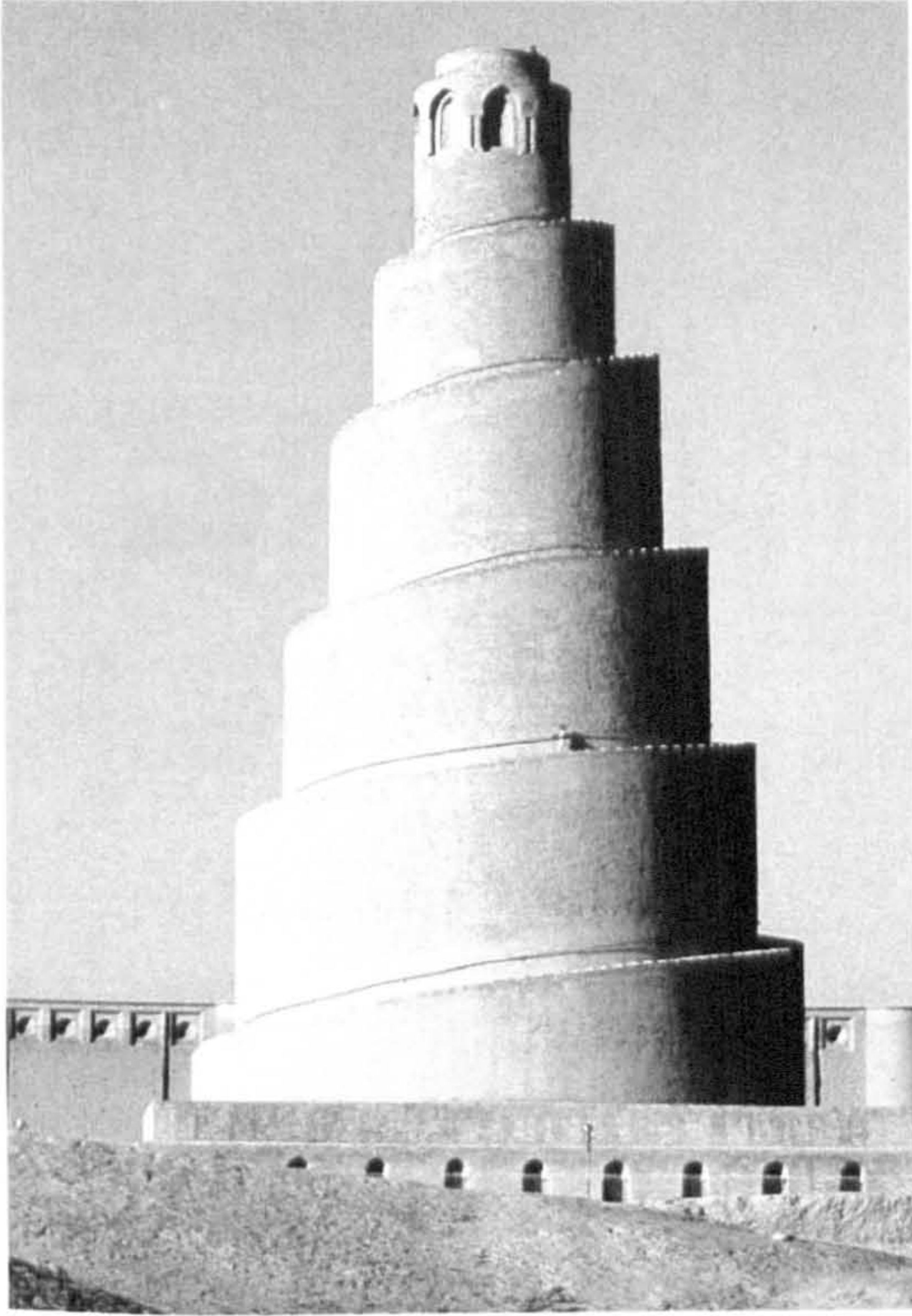
Fig 2.8 Spiral minaret, Samarra (from The Threat to World Heritage 2003 )
