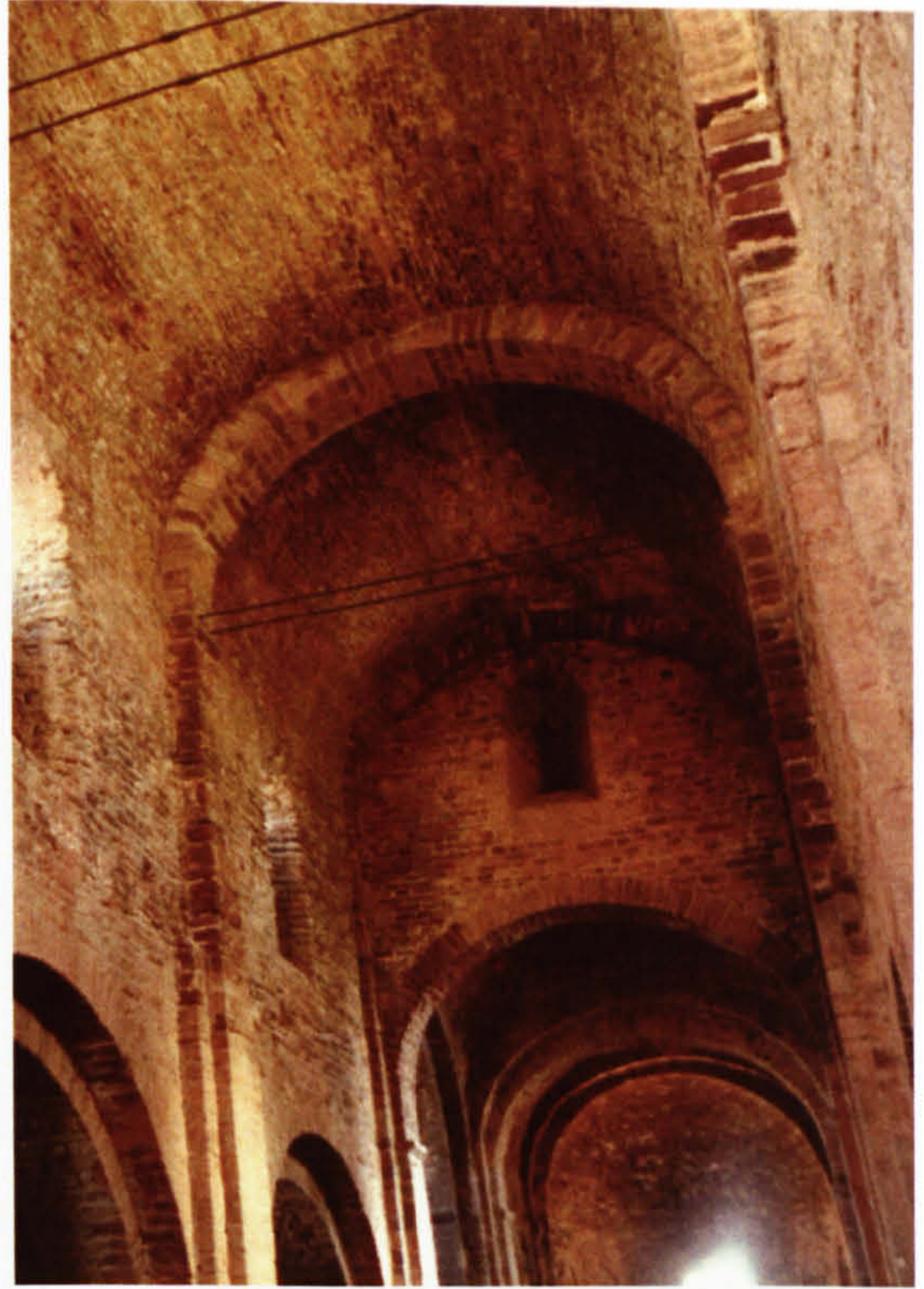
Fig 6.2 Nave vault and clerestory (courtesy of Peter Reed)
