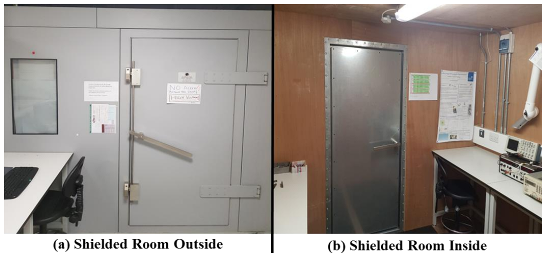
Figure 81: Shielded grounded metal room acting as a Faraday cage.
